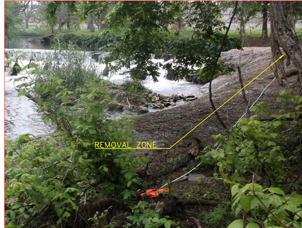
DEFICIENT STRUCTURE 2. CONCRETE BANK-STABILIZATION STRUCTURE
