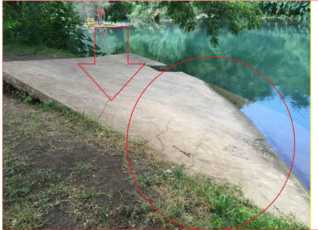
DEFICIENT STRUCTURE 1. CONCRETE BANK-STABILIZAION STRUCTURE
