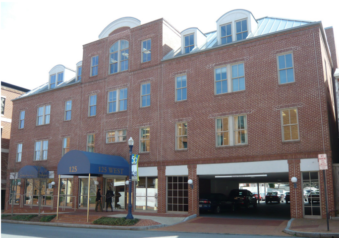
Window design includes vertical proportions (in pairs) and true divided lights
