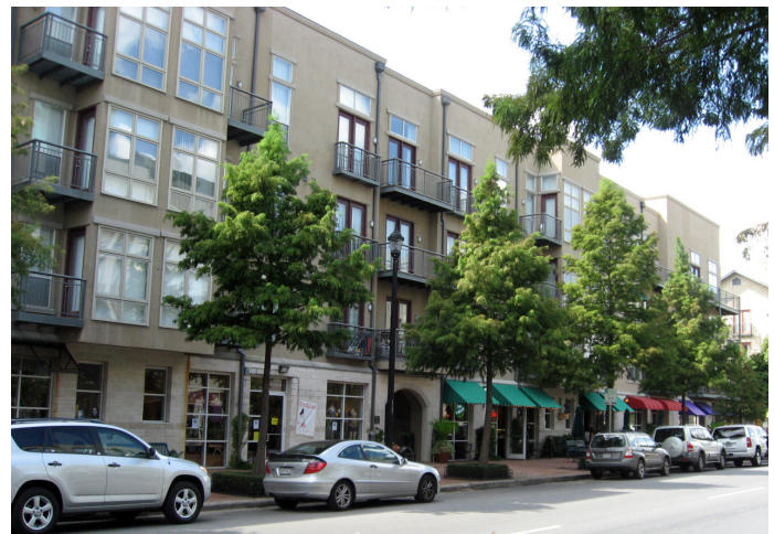
Awning / Canopies, Cornice; Balcony
