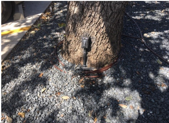
Poor Example: Drip irrigation wrapped around the tree trunk of an established tree. Water applied on the tree trunk and root flare can introduce disease and decay; restrict tree diameter growth and possibly lead to tree mortality.
