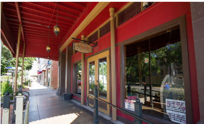
Retain cast iron column ( 127 E Hopkins St)
