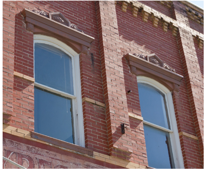
Pressed metal window hoods (101 E Hopkins St)
