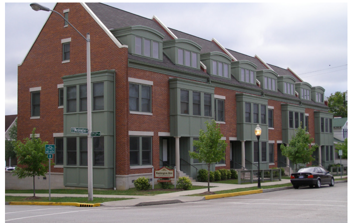
Change in Materials; Cornice; Stoop
