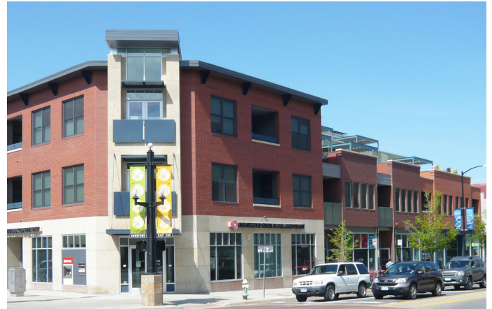
Wall Notches; Change in Materials (first floor); Cornice
