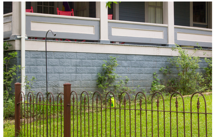
Pressed metal skirting (323 Scott St)
