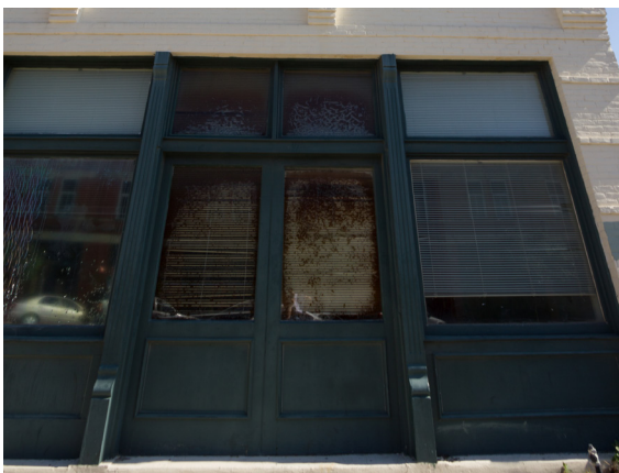
Retain cast iron storefront (102 N LBJ Dr)
