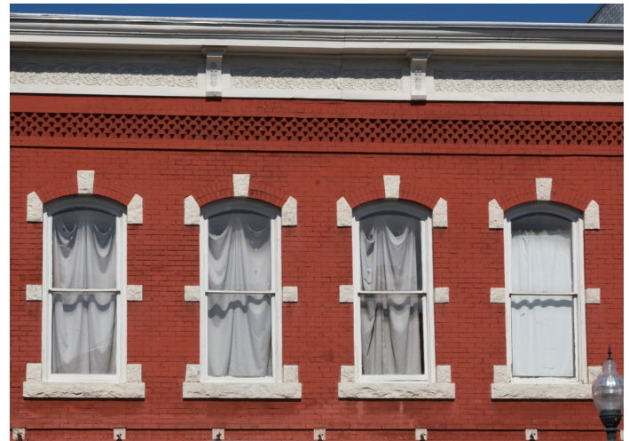
Clear glass in windows (125 N Guadalupe St)
