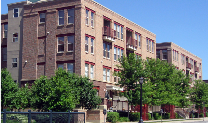
Vertical Expression Lines; Cornice; Balcony
