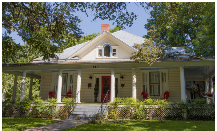
Porch is elevated (810 W San Antonio St)
