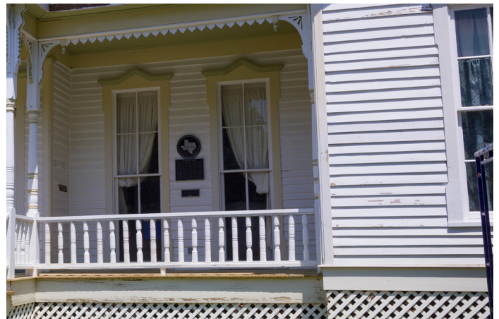
Horizontal wood siding is the most common exterior wall surface (716 W Hopkins St)
