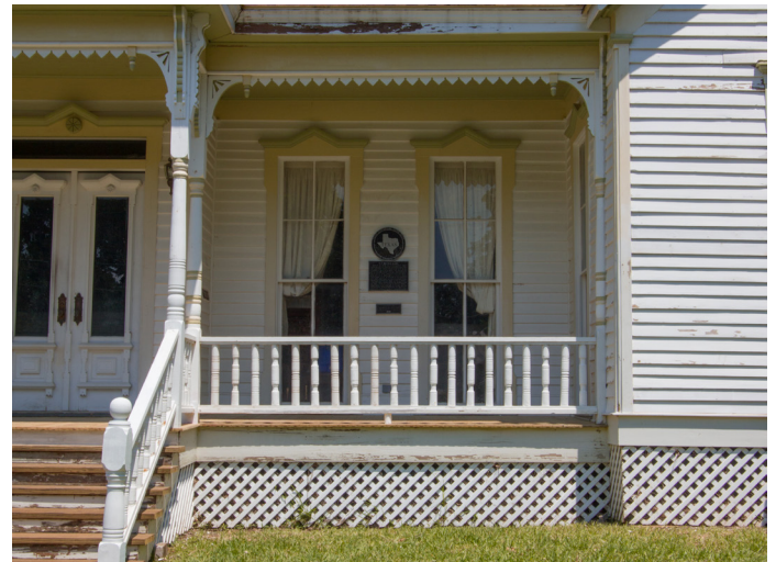
Wood lattice skirting (716 Belvin St)
