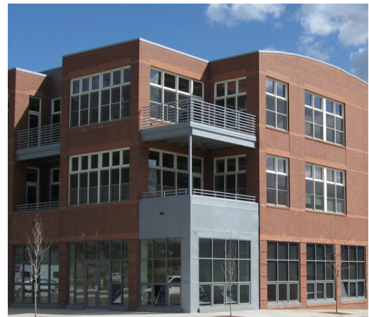
Varied Upper Floor Heights; Wall Offsets; Cornice
