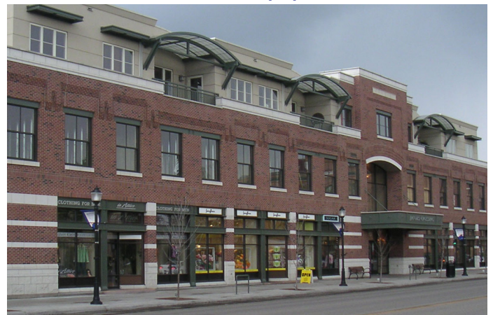
Cornice; Change in Materials (upper floor); Window Design includes insets, sills, and true divided lights
