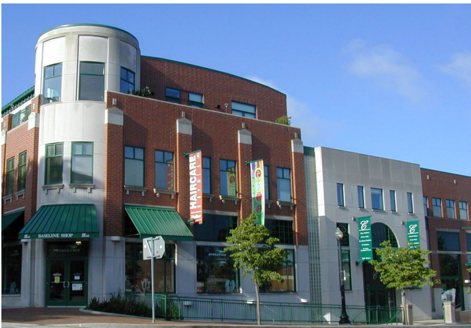
Varied parapet line; Change in Materials, Vertical Expression Line (pilasters)
