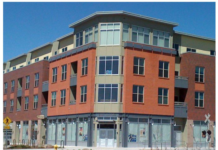
Wall Notches; Change in Materials (vertical and horizontal); Cornice
