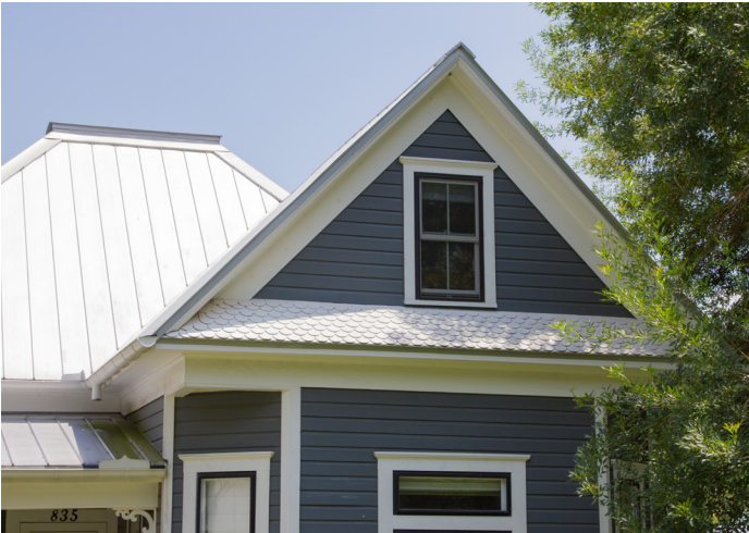
Roof Form (835 W Hopkins St)
