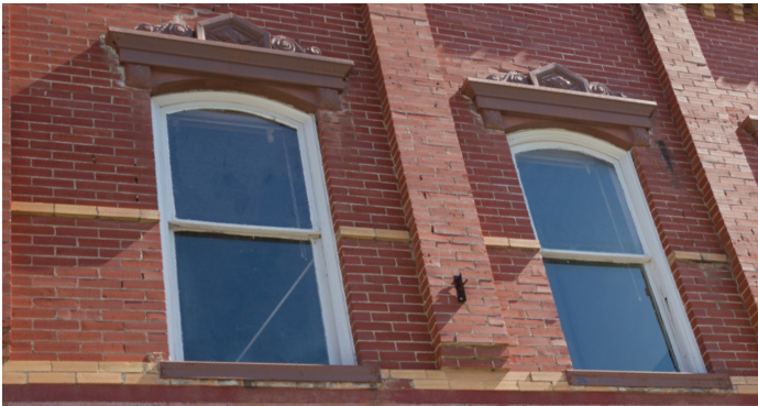
Retain wood windows (101 E Hopkins St)
