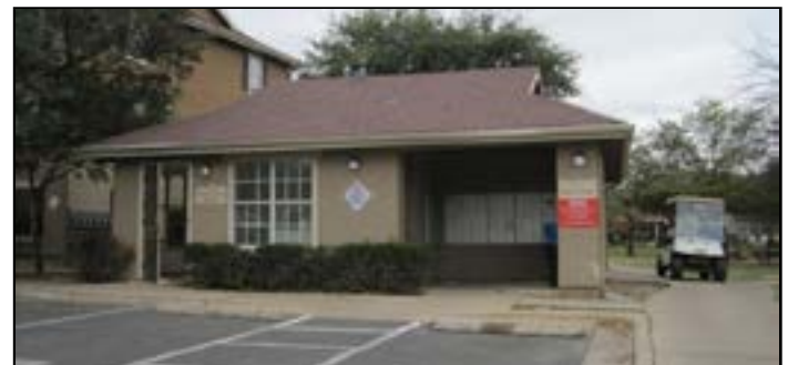
Weather-protected shelter with material and design that are consistent with the primary structure which has clear pedestrian access: appropriate
