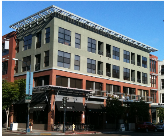
Horizontal expression: cornice, molding at second story and change in materials Cornice; Second-Floor-Expression-Line
