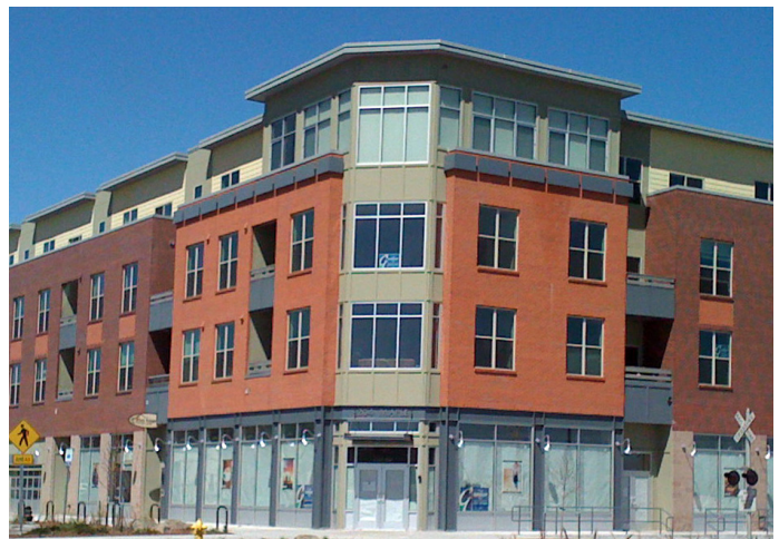
Vertical expression: Wall Notches, Change in Materials; Varied Massing: Stepback at upper floor Wall Notches; Change in Materials (vertical and horizontal); Cornice
