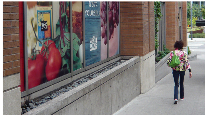
Integrate the elements of a building facade to respond to changes in topography.
