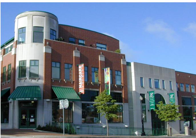
Vertical expression: pilasters, wall notch and material changes that reflect traditional modules. Varied-parapet line; Change in Materials, Vertical-Expression-Line (pilasters)
