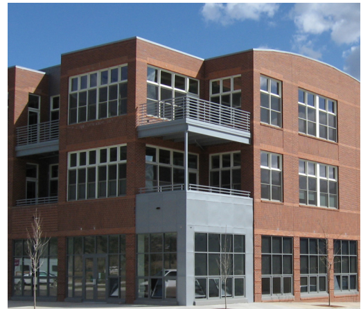
Vertical expression: changes in material and color, wall notches Varied Upper Floor Heights; Wall Offsets; Cornice
