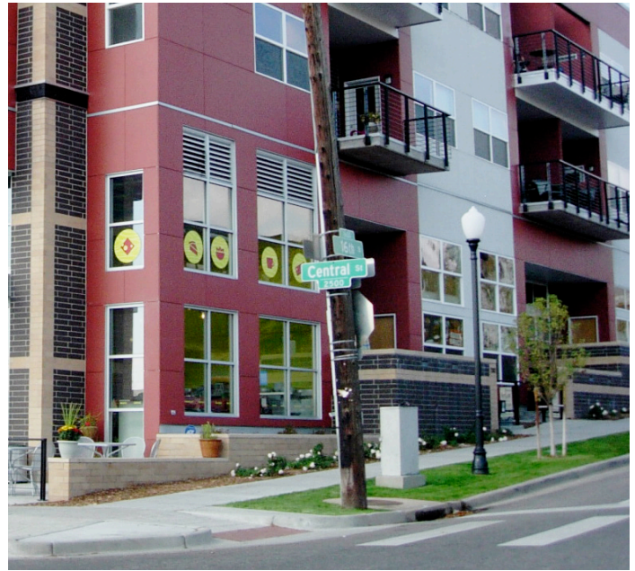
Design a building to step with the existing topography of a site.
