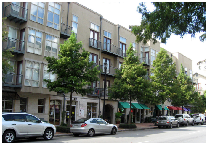
Awning / Canopies, Cornice; Balcony
