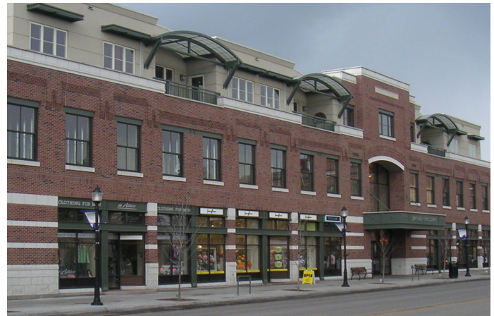
Horizontal expression: cornice line, window sills, and accent materials. Cornice; Change in Materials (upper floor); Window-Design includes insets, sills, and true divided lights
