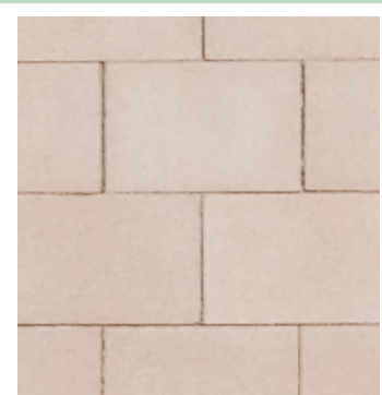
Finished Ashlar Stone
