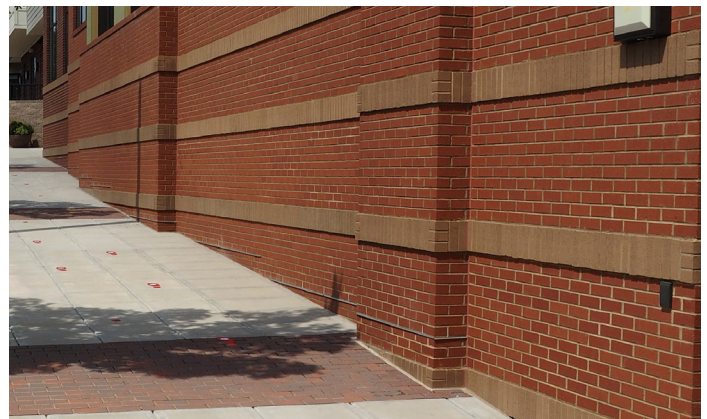
This image is inappropriate because a pedestrian scaled is not maintained.
