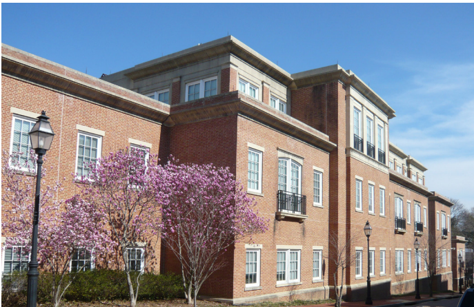
Varied Massing: Upper Floor Stepback; Wall offset as vertical expression Varied Upper Floor Massing; Wall Offset; Cornice
