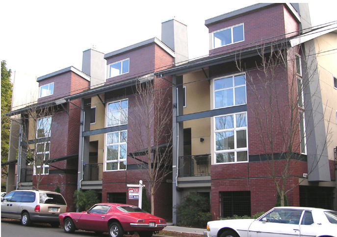
Wall Offset; Cornice
