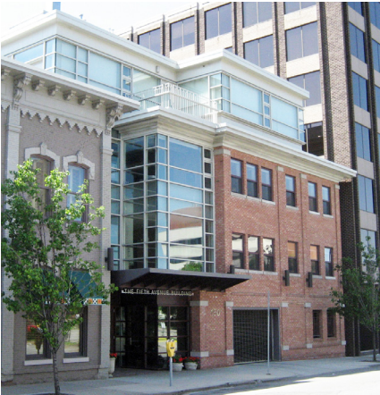
Step down in height adjacent to historic building
