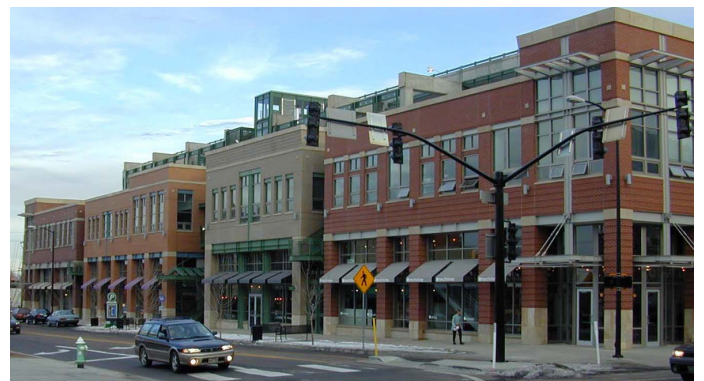
Wall Notch; Awning / Canopy; Window moldings at second floor; Cornice
