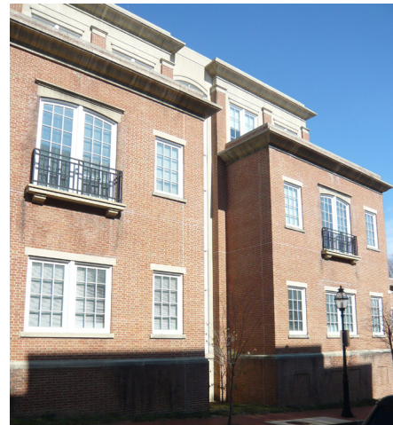
Varied Upper Floor Massing; Wall Notch; Cornice
