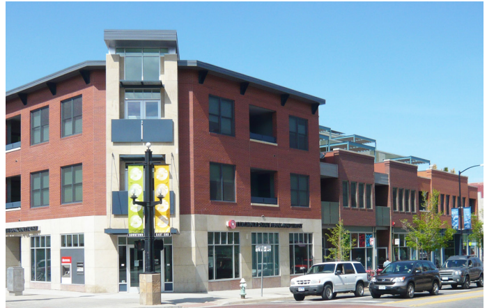
Vertical Expression: Wall notches and changes in color Wall-Notches; Change in Materials (first floor); Cornice
