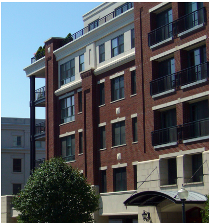
Vertical Expression Line (pilasters or attached columns); Cornice; Change in Material (first and upper floors)
