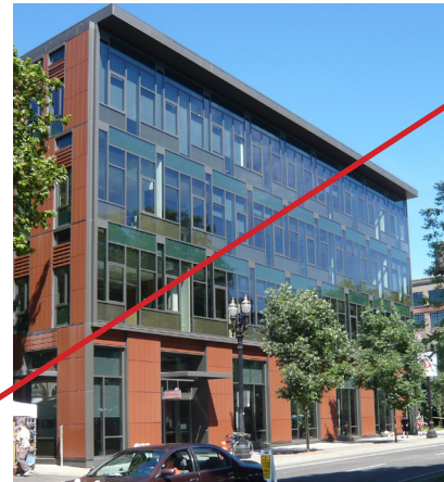
Change in Materials (at first floor); Cornice; Window design includes vertical proportions
