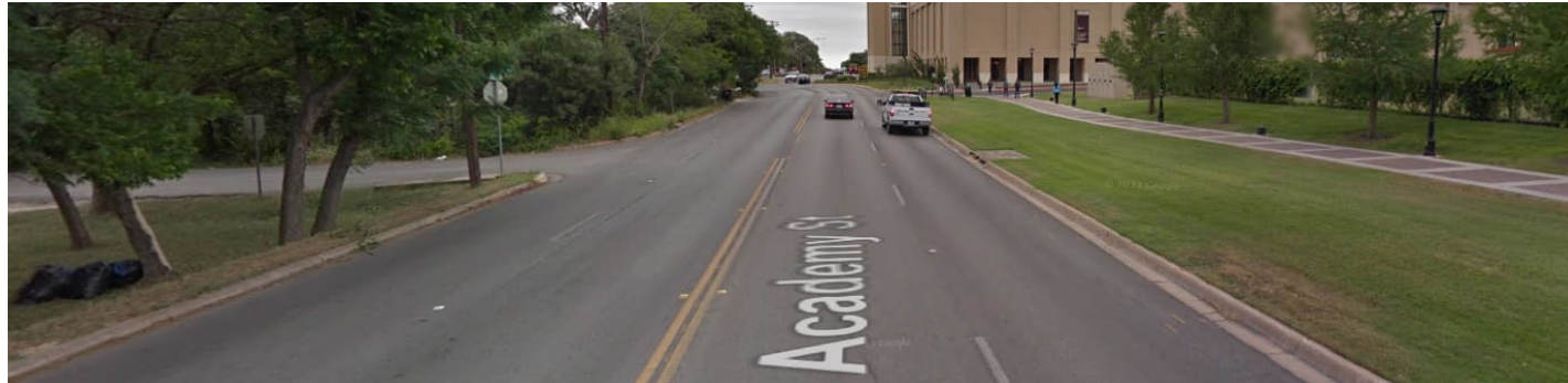
Previous Striping (No Traffic Calming Measure)
