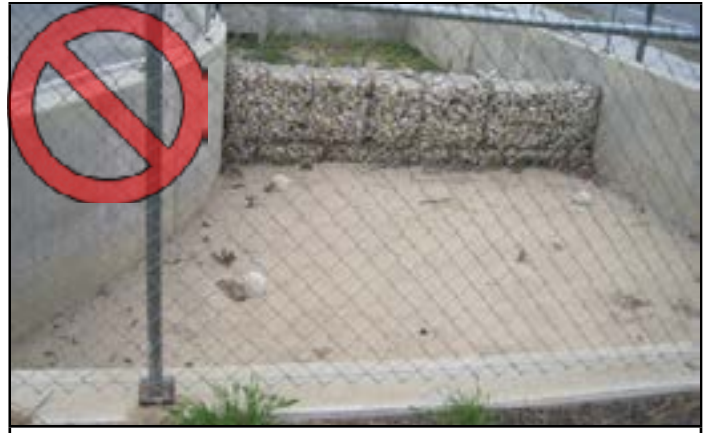
Rectangular facility with concrete walls fenced and built at the street edge: inappropriate
