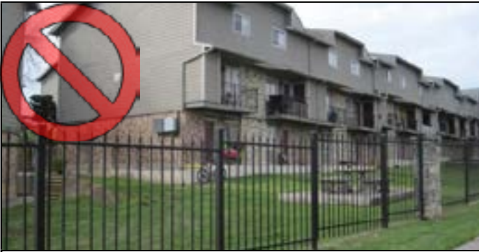
Unarticulated perimeter fence: inappropriate
