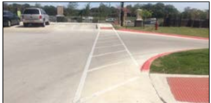
Pedestrian crosswalk distinguished from the driving surface via painted striping: appropriate
