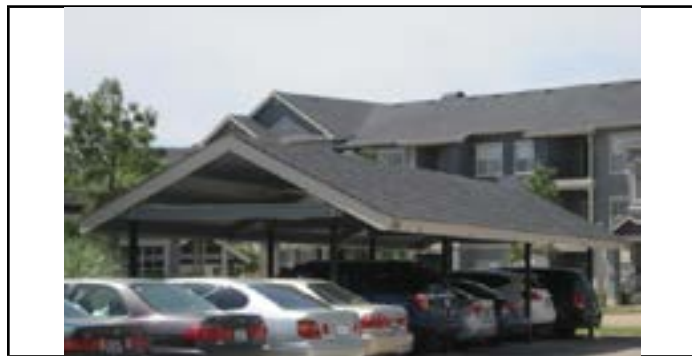
Carports complement the building in terms of materials and trim: appropriate
