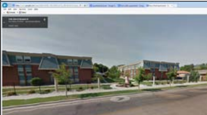
Perimeter fence which is more than 50% transparent with masonry columns and pedestrian access: appropriate
