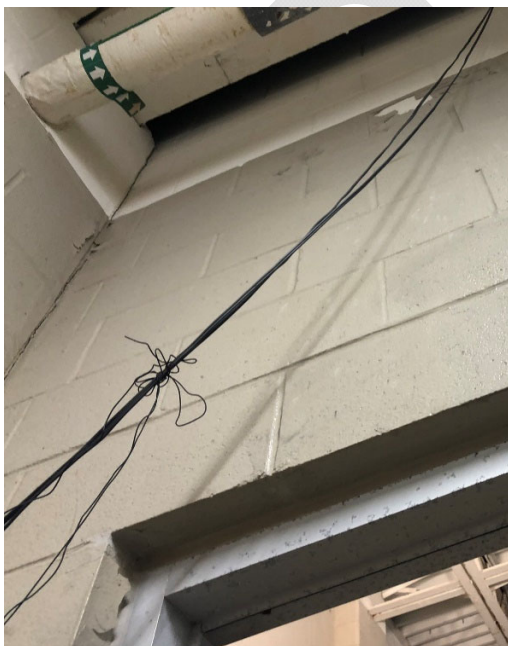
Wiring is exposed, unprotected and generally messy.
