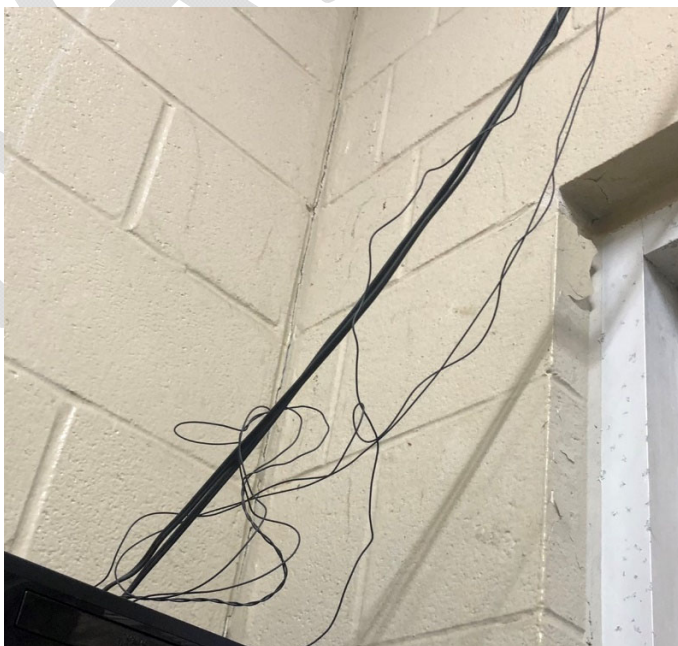
Wiring is exposed, unprotected and generally messy.
