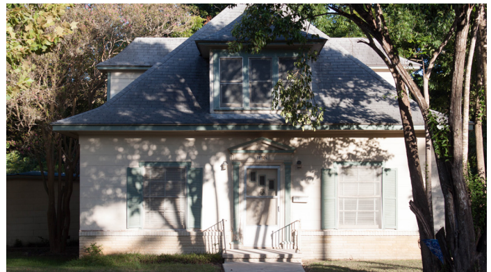
Asbestos shingles were used in the 1930s and 1940s as siding (1107 W San Antonio St)
