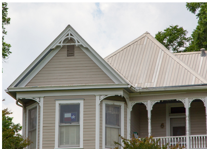
Victorian house has a simple gable roof and ornate details at the minor roof forms (724 Burleson St)
