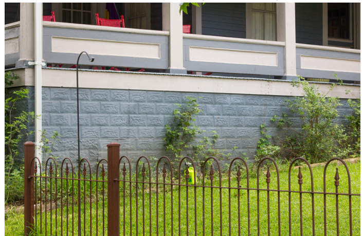
Pressed metal skirting (323 Scott St)
