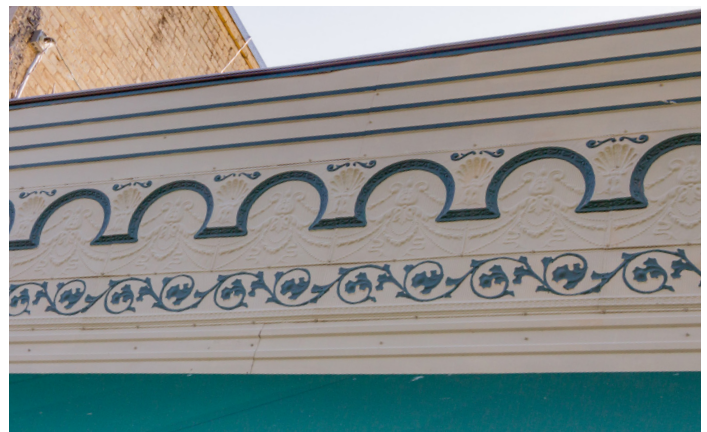
Pressed metal cornice - modified but retains scale (114 N LBJ Dr)
