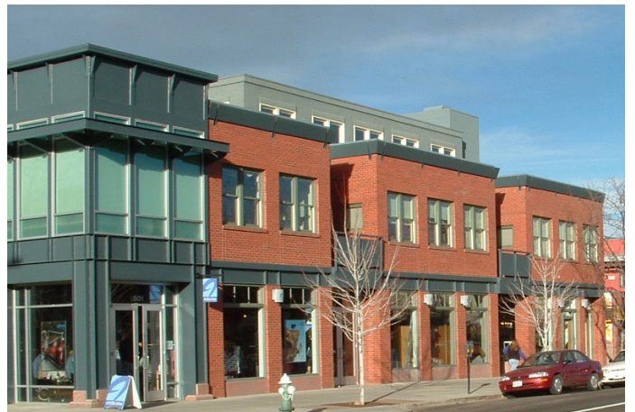
Wall Notch; Horizontal Expression Line
