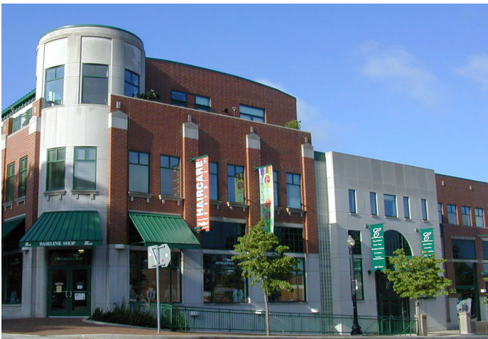
Vertical expression: pilasters, wall notch and material changes that reflect traditional modules
