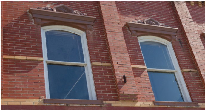
Retain wood windows (101 E Hopkins St)
