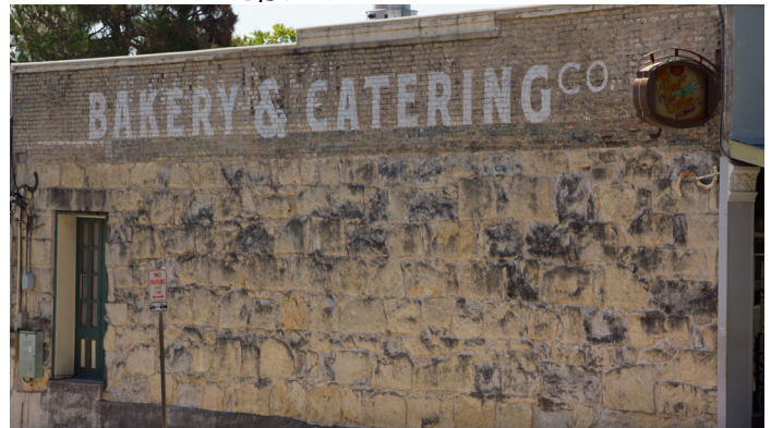
Cut stone blocks for walls of older buildings (142 N LBJ Dr)
