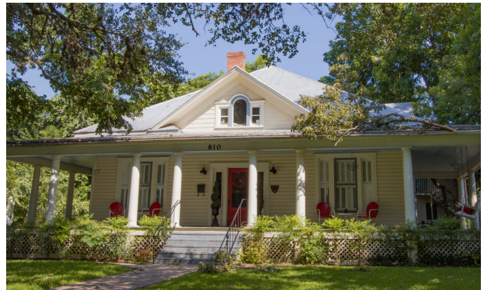
Porch is elevated (810 W San Antonio St)
