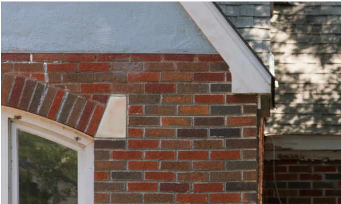
Brick with stone accents (727 W Hopkins Street)
