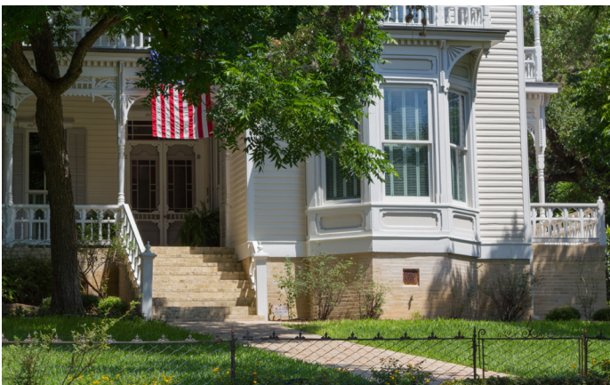
Brick perimeter wall supports house (832 Belvin St)
