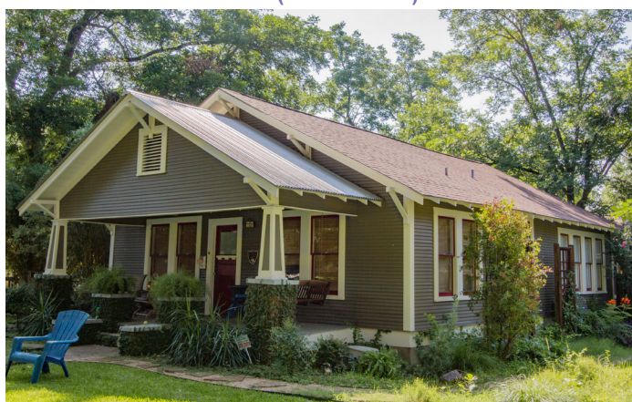
Simple gable roof is found on Craftsman houses (811 W San Antonio St)
