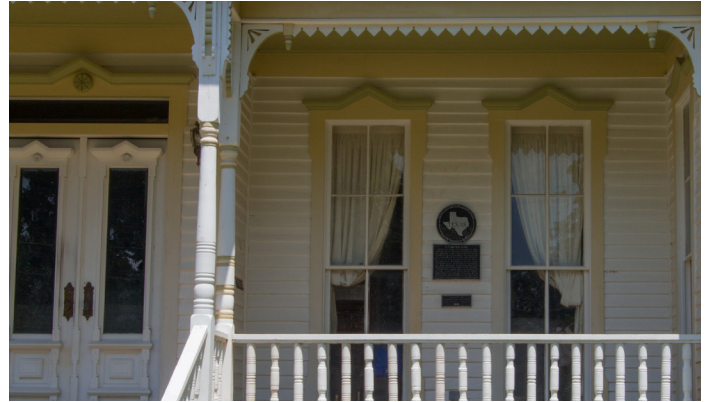
Tall narrow openings and glass in the sash help to establish a date of the house (716 Belvin St)
