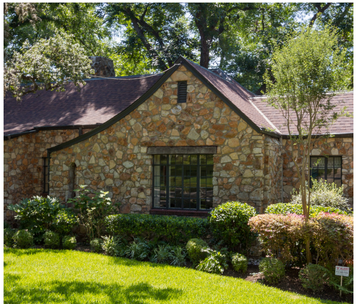
Historic application with stone exterior (809 Belvin St)
