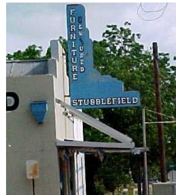
Poor Example - sign extends above the building roof
