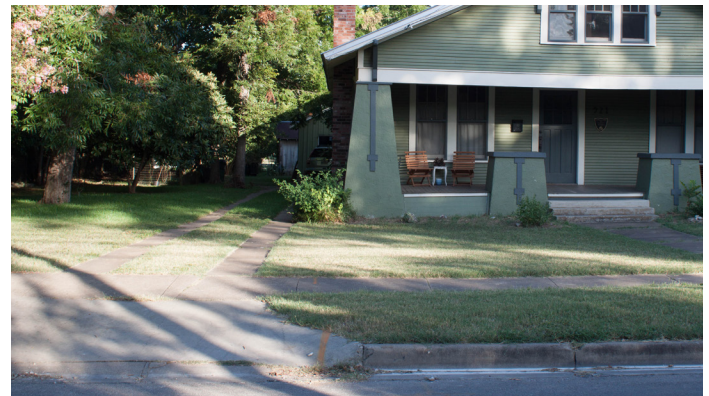
Concrete ribbons leading to garage behind the house (921 W San Antonio St)
