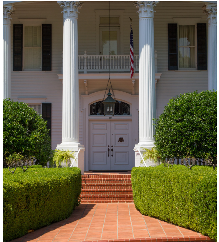
The entry doors and transom are in scale with the ground entry porch (227 N Mitchell Ave)
