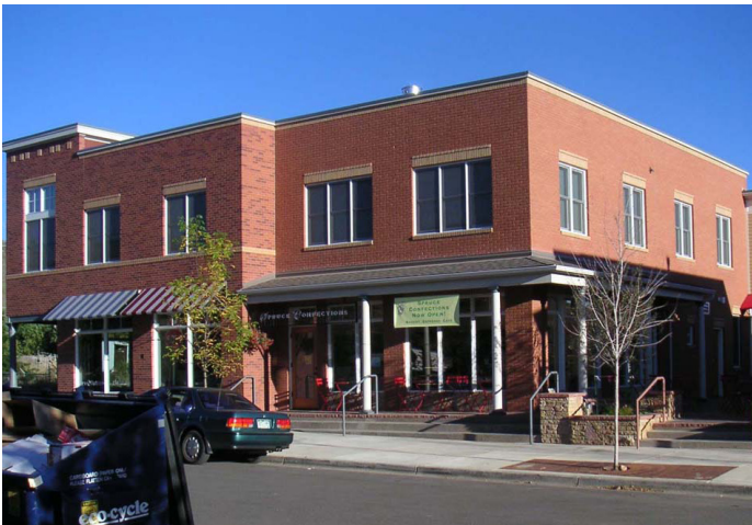
Wall Offset; Vertical Window Proportions
