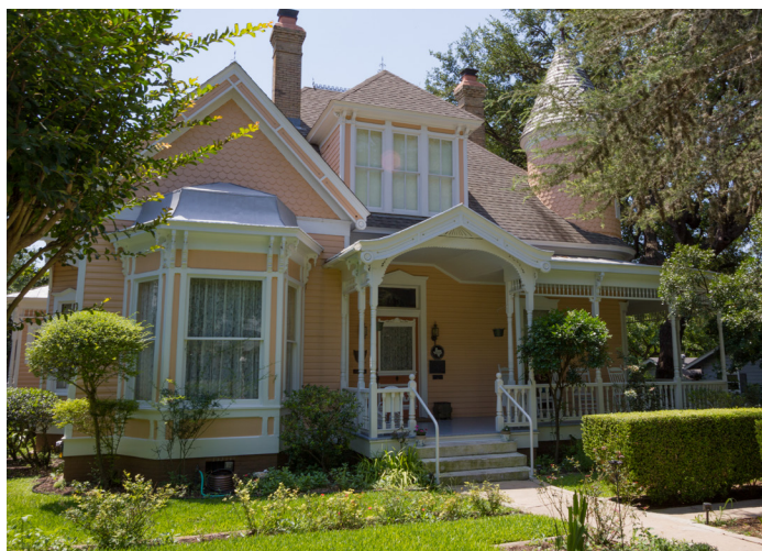
Complicated roof form and elaborate details indicate Queen Anne (727 Belvin St)
