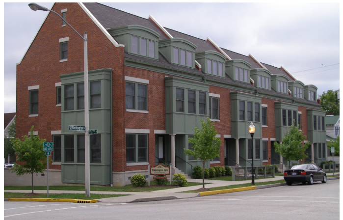
Change in Materials; Cornice; Stoop
