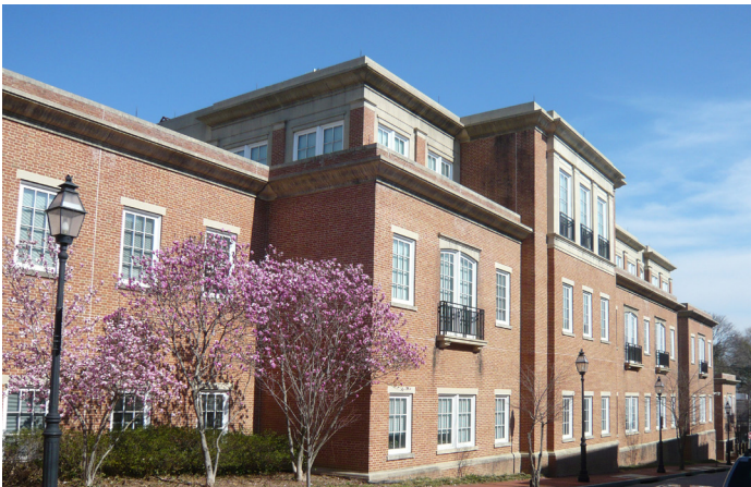
Varied Massing: Upper Floor Stepback; Wall offset as vertical expression
