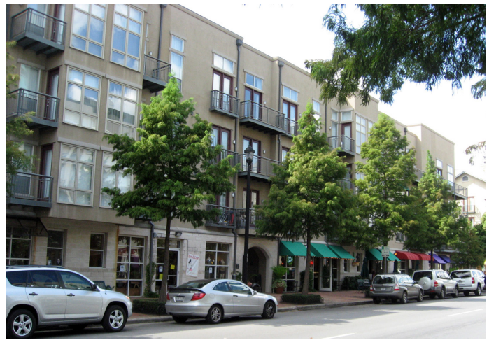
Awning / Canopies, Cornice; Balcony
