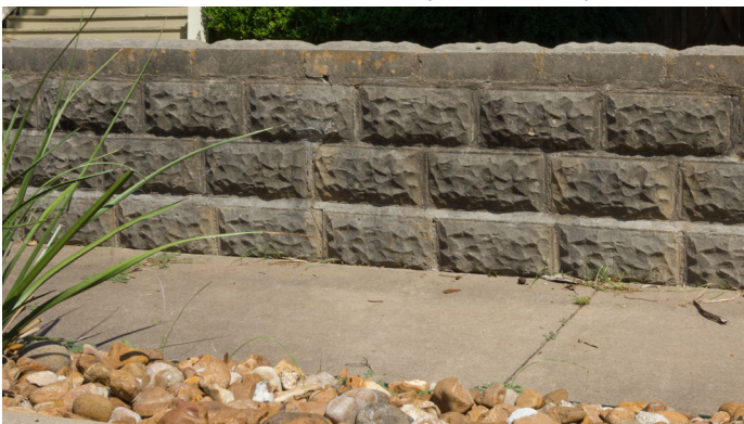
Rough faced concrete block (1024 W San Antonio St)
