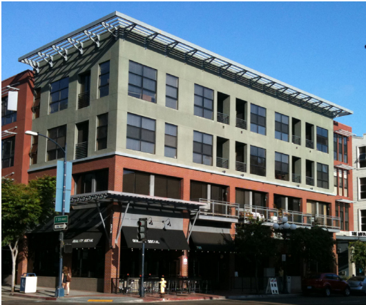
Horizontal expression: cornice, molding at second story and change in materials
