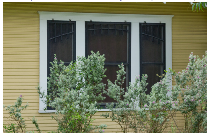
Window screens with detail appear on Craftsman and Prairie style houses (620 Rogers St)
