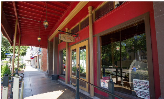
Retain cast iron column (127 E Hopkins St)
