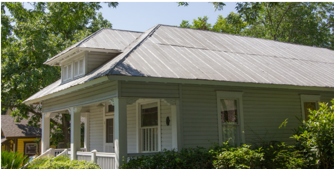
One of many standing seam metal roofs in San Marcos (221 Johnson Ave)
