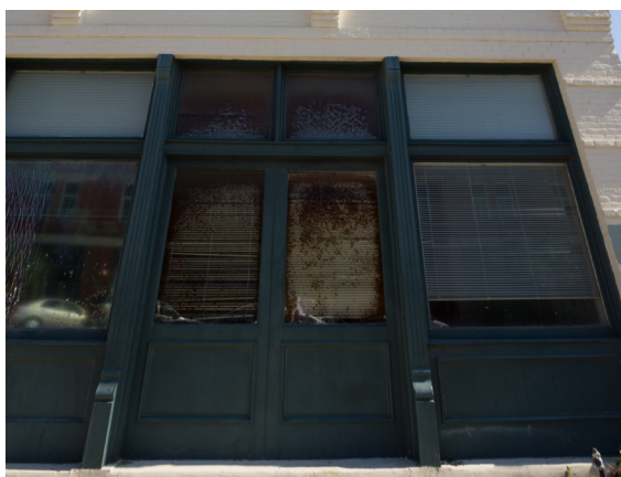
Retain cast iron storefront (102 N LBJ Dr)
