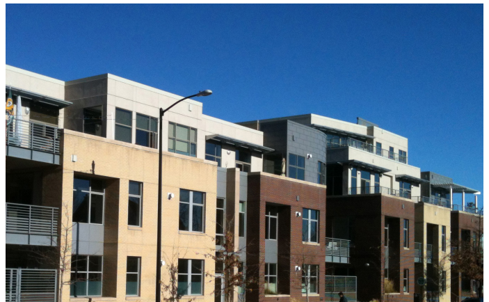
Wall Offset; Horizontal Expression Line; Materials Change
