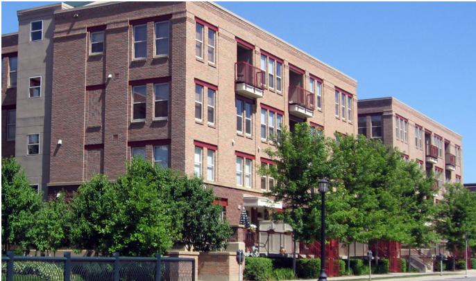
Vertical Expression Lines; Cornice; Balcony
