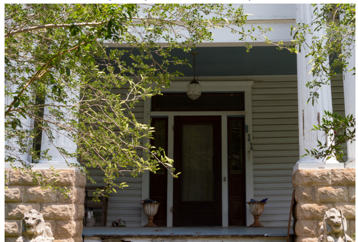
Single entry door surrounded by transoms and side lights (811 W Hopkins St)
