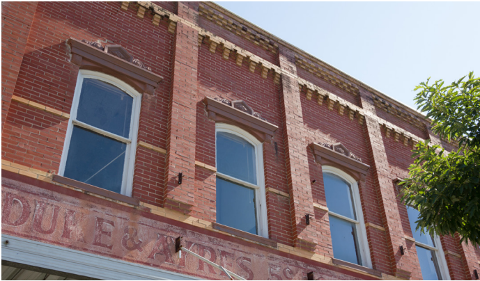
Brick cornice / Brick banding (101 E Hopkins St)
