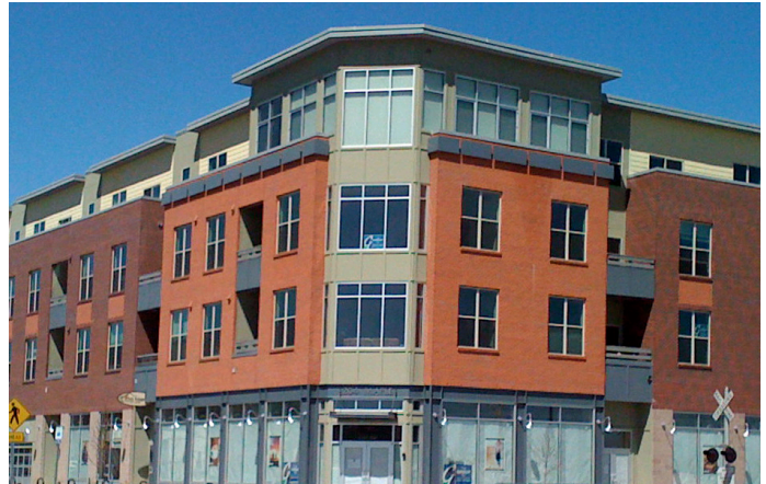
Vertical expression: Wall Notches, Change in Materials; Varied Massing: Stepback at upper floor
