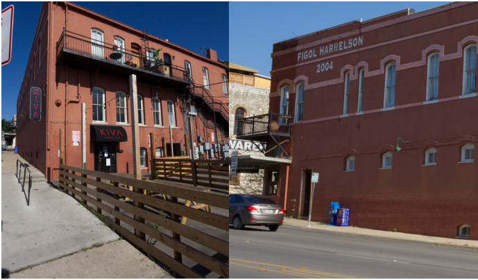
“New” rear entrance and original entrance along Hopkins Street (202 N LBJ Dr)
