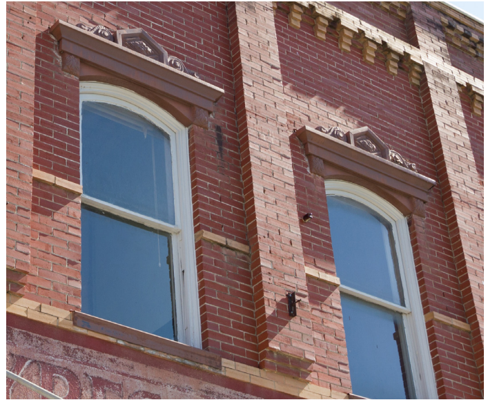
Pressed metal window hoods (101 E Hopkins St)
