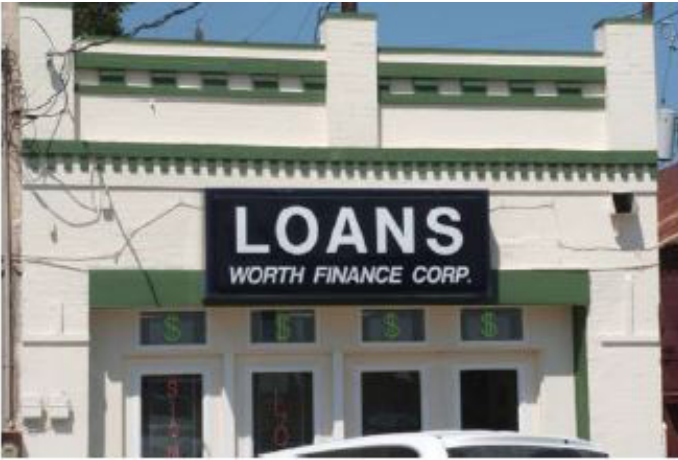
Poor Example - this sign is out of scale with the building and covers details.
