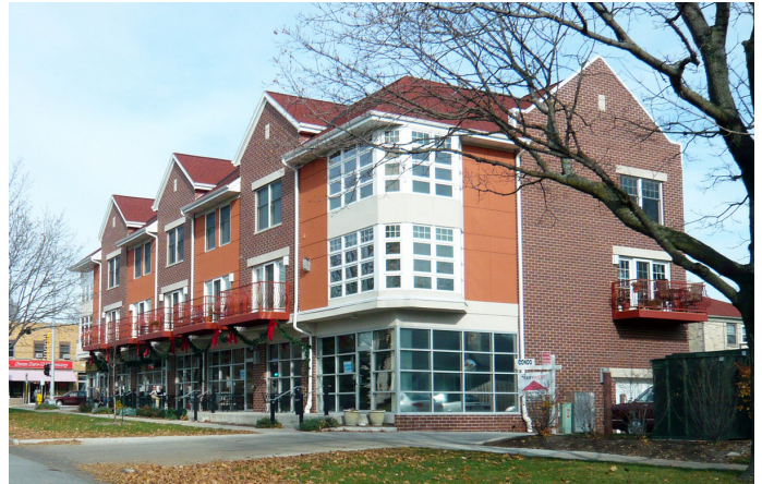
Varied Upper Floor Massing; Change in Materials; Balcony
