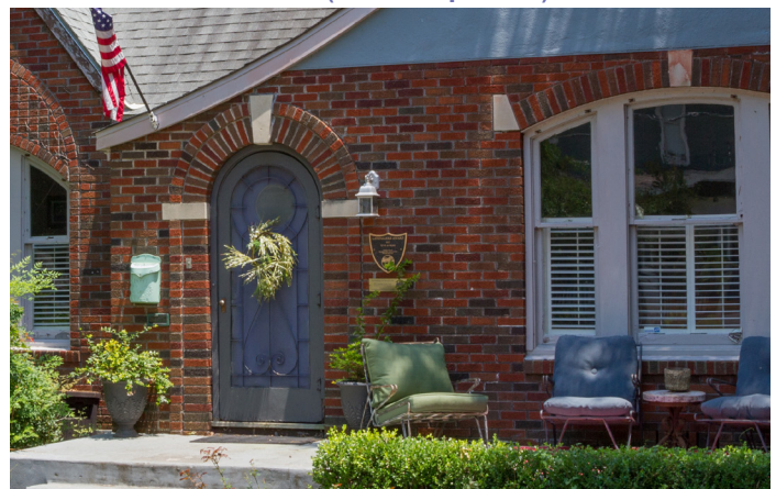
Retain original wall surface to retain character (727 W Hopkins St)
