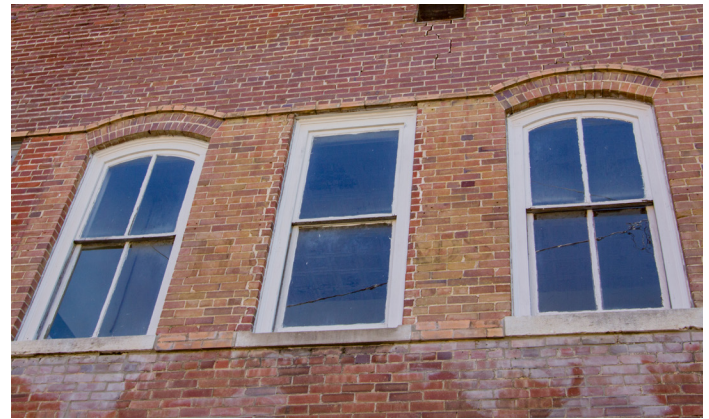
Retain wood window frame and sash (101 E Hopkins St)
