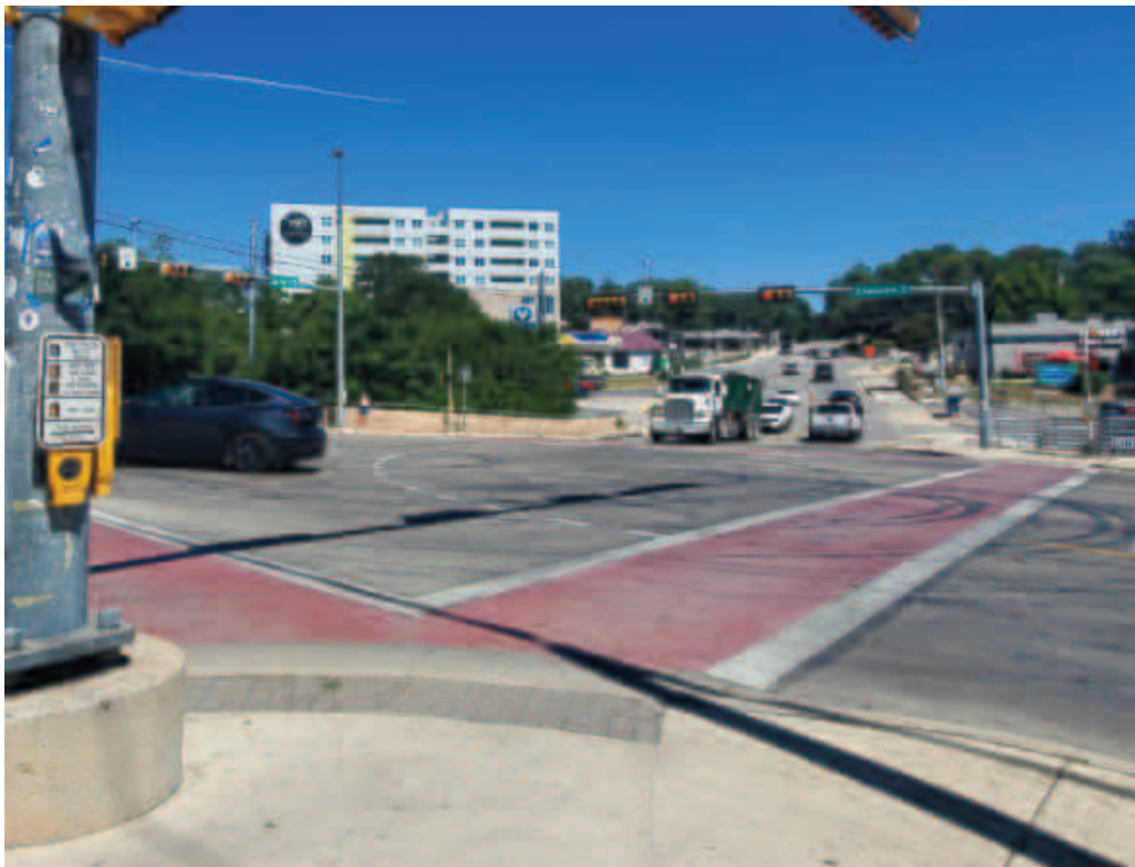
Crosswalks, used by pedestrians, at the approximately 80 ft. wide portion of Sessom Drive at the intersection of North LBJ Drive and Sessom Drive.
