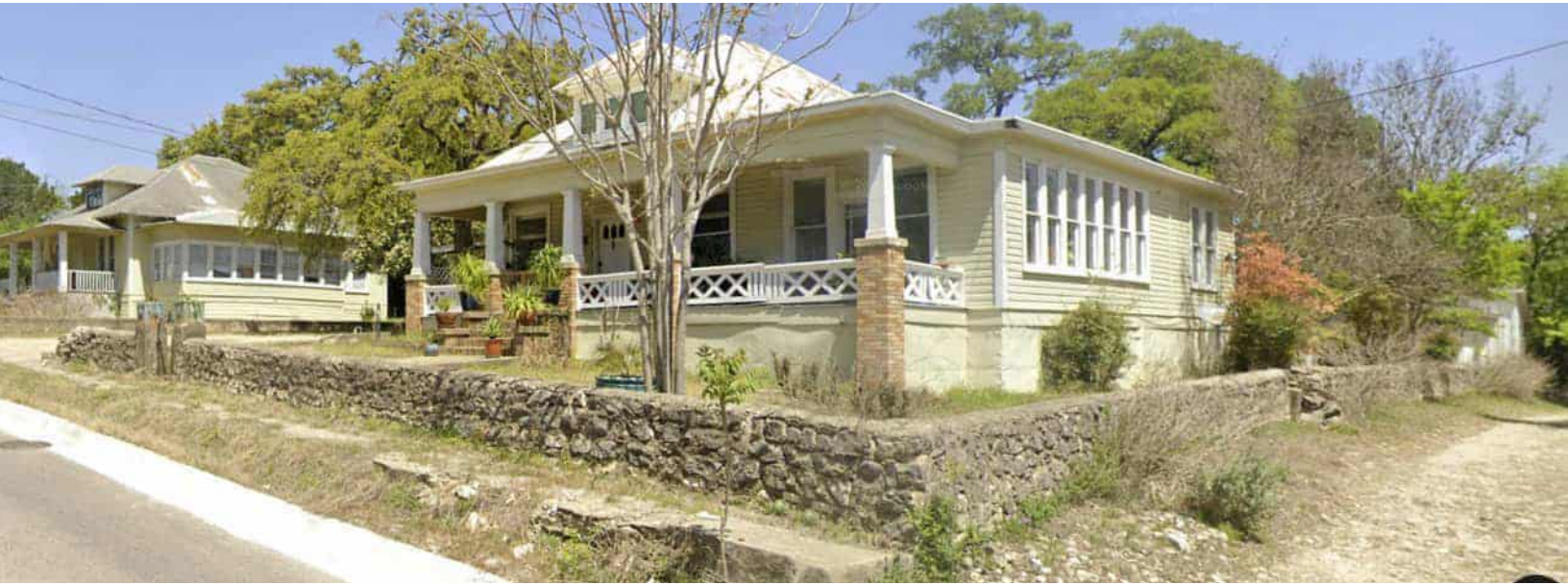
The existing home at 918 Chestnut Street is apart of the Park Addition plat and is eligible for the National Register of Historic Places.
