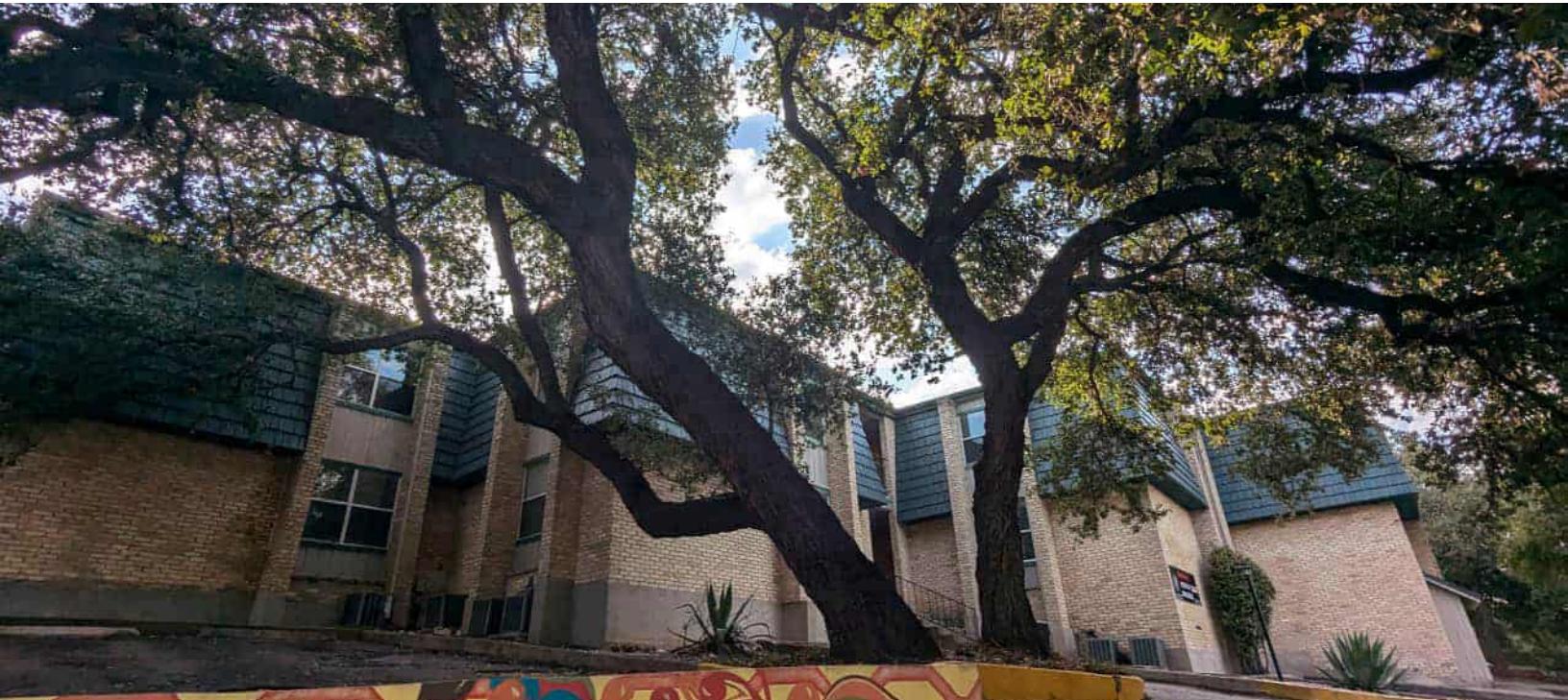
810 North LBJ Apartments, highlight the steep elevation changes in the Plan Area.
