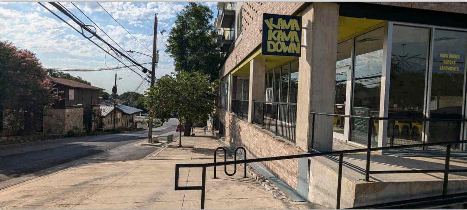
Vie Lofts commercial space fronting on Chestnut Street. 817 Chestnut Street.
