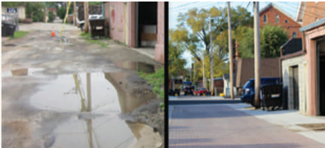
Figure 2: Example from Dubuque, Iowa of a green alleyway conversion. Source: The San Marcos Green Alley Initiative
