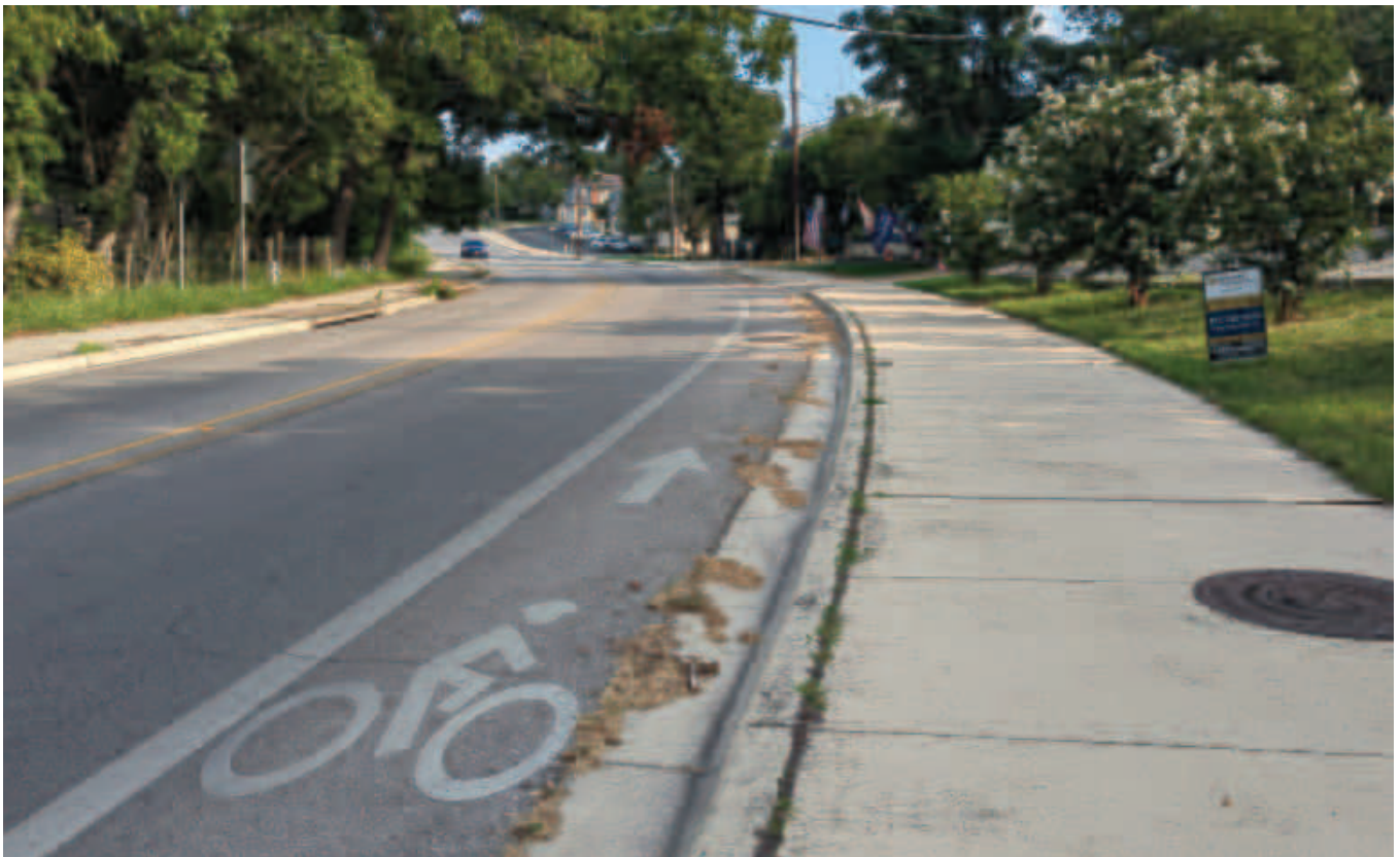
View of North LBJ Drive. 5 ft. sidewalks constructed in 2015 and bicycle facilities on one side.
