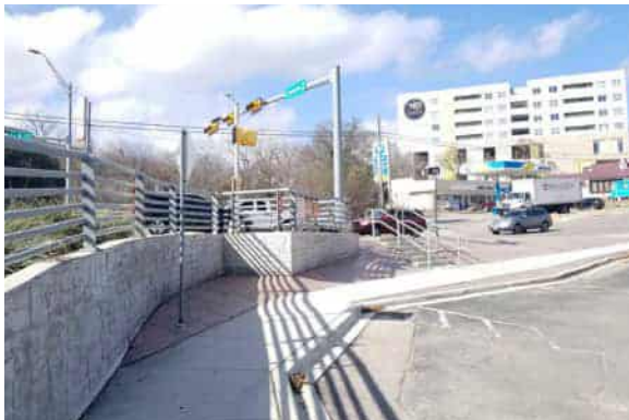
Street improvements at Sessom Street bordering 700 N. LBJ Drive.
