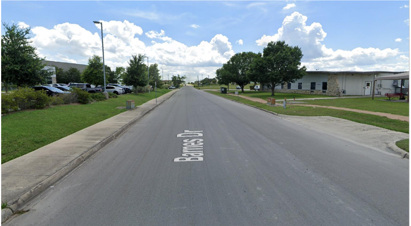
Barnes Dr. at rear of Mensor facility, facing south
