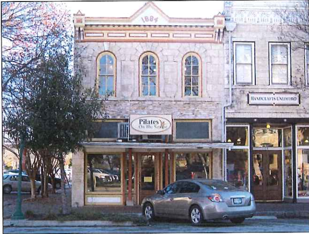
Leave natural masonry finishes unpainted when feasible.
