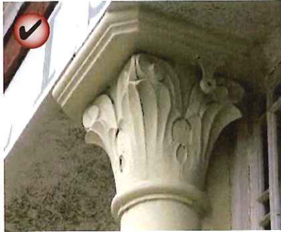
Maintain protective coatings, such as paint, on exposed metals.
