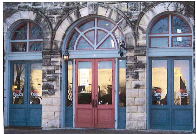
Bright colors can be used to identify a building entrance.
