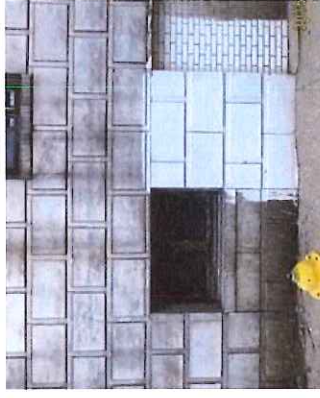
[1] A test patch should always be done before using a chemical cleaner to ensure that it will not damage historic masonry, as in this instance, terra cotta.
