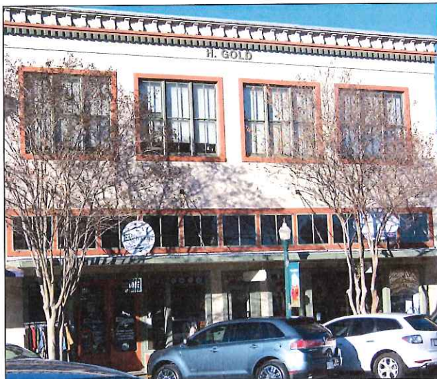
Choose colors for trim, accents, and architectural details that complement the main color on the body of the structure.
