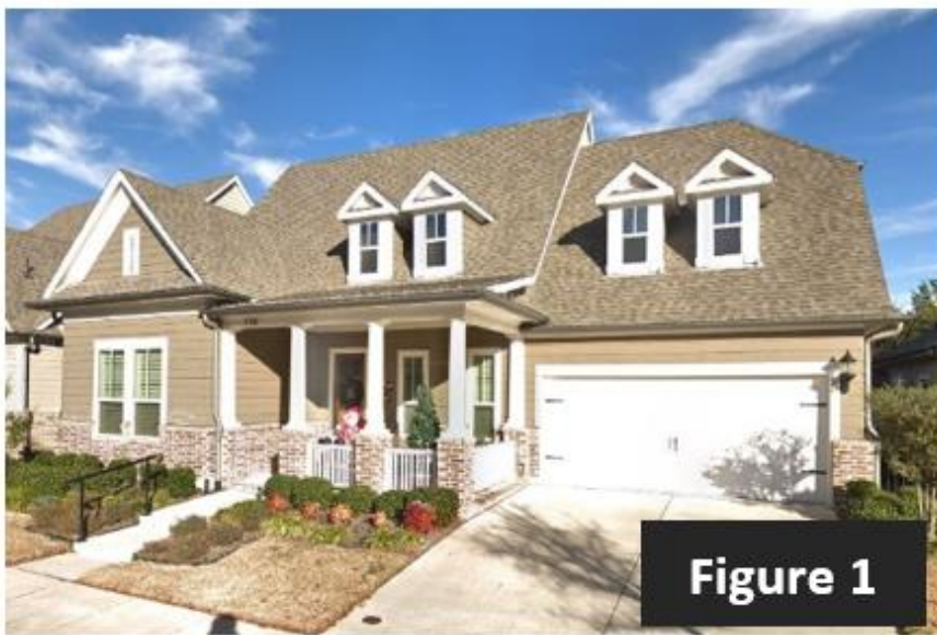
Garage is set-back from front wall plane and porch
