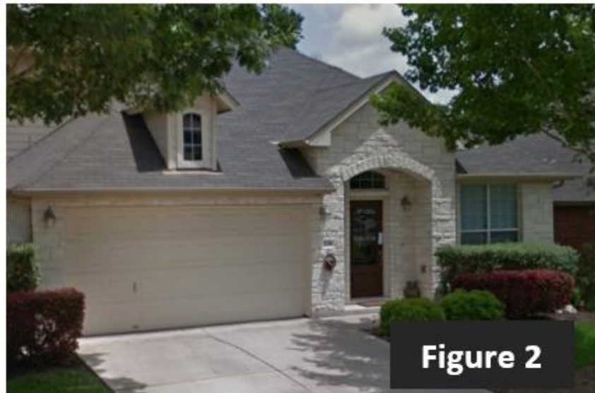
Garage is flush with front wall plane
