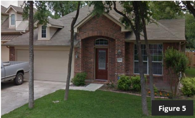
Entry door is flush with facade
