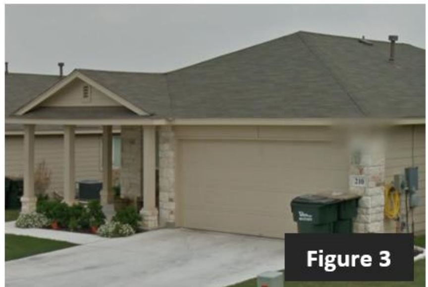
Garage is flush with porch
