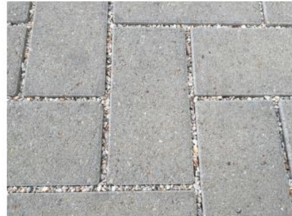
FIGURE B.4.7 EXAMPLE OF PICPS IN A HERRINGBONE PATTERN. San Marcos, Texas. Source: Tetra Tech.
