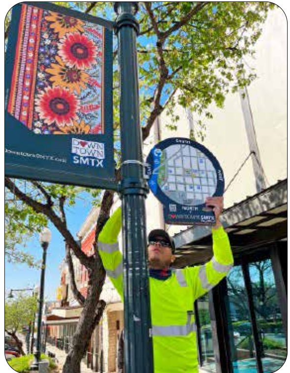
Wayfinding signs being installed Downtown (COSM)
