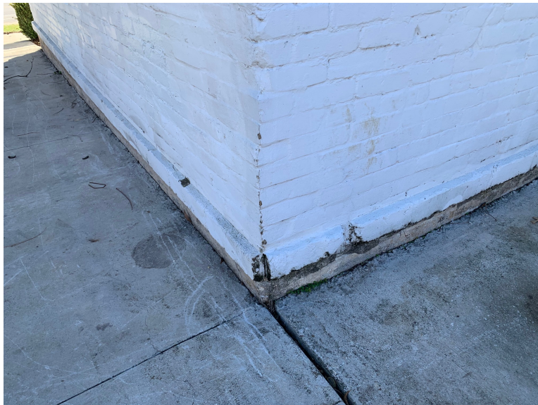
The Calaboose is constructed of machine-cut bricks on a poured concrete foundation, typical of construction between 1912 and 1922.
