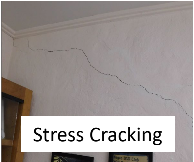
Foundation Cracking
