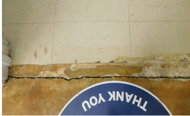
Foundation Cracking
