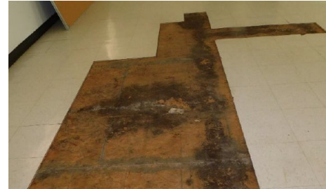
Subfloor Water Damage
