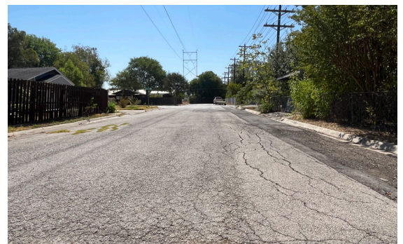
Cracked asphalt along Highline Drive.
