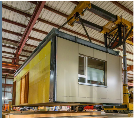
One “block” of a MiCASiTA modular home under construction. This component can become a 576-square foot standalone home, or multiple blocks can be combined to form a larger structure.
