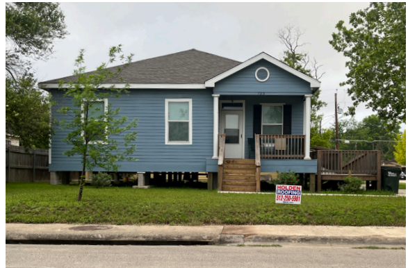
Single-story home on Sturgeon Drive, raised to meet floodplain development requirements.
