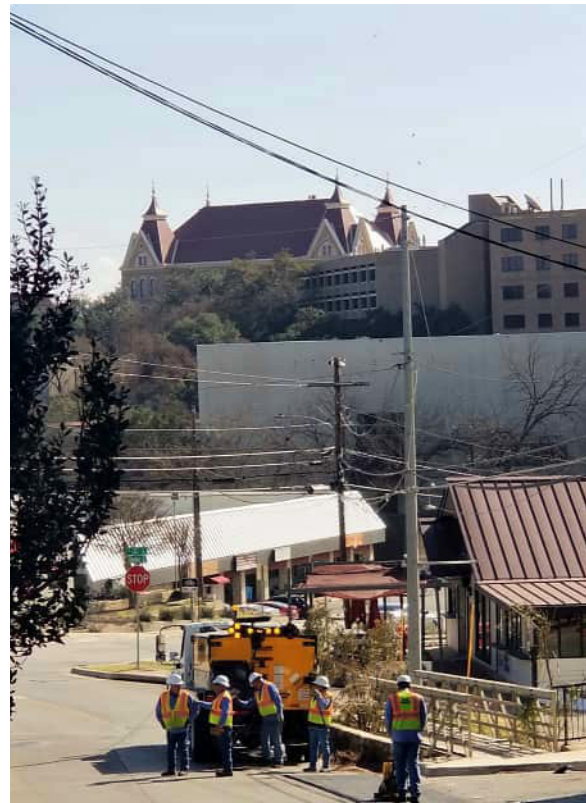
COSM staff making repairs at Chestnut Street and North LBJ Dr.
