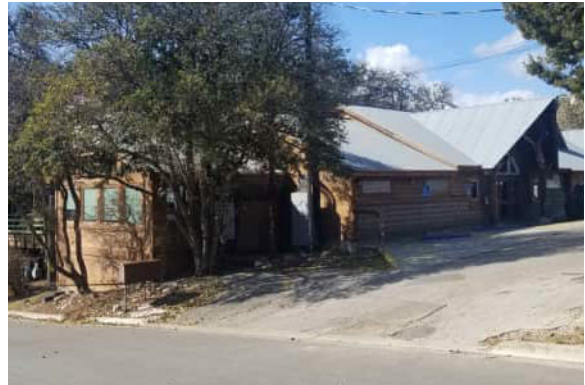
View of Grins Restaurant on Forest Street.
