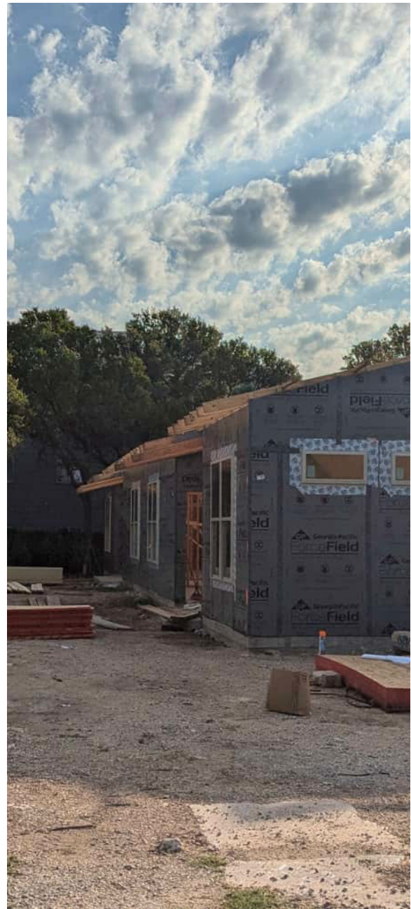
Duplex construction at 1106 Chestnut Street.
