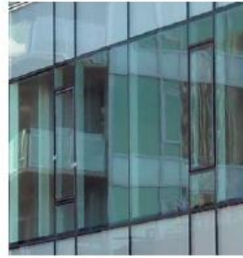
Glass Curtain Wall
