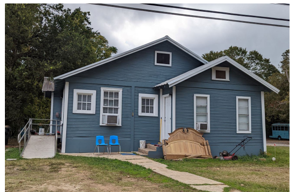
Single-family home with side-facing entryway.
