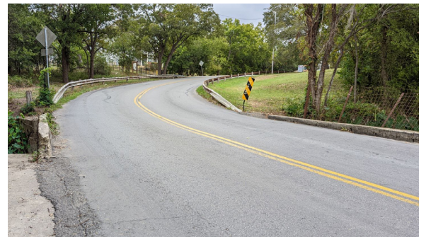
Lack of sidewalks along Cape Road.
