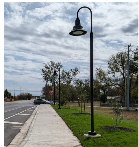
Pedestrian-scale street light on River Road installed in the summer of 2024. The wide lampshade directs light downward, which is a standard of the International Dark Sky guidelines.
