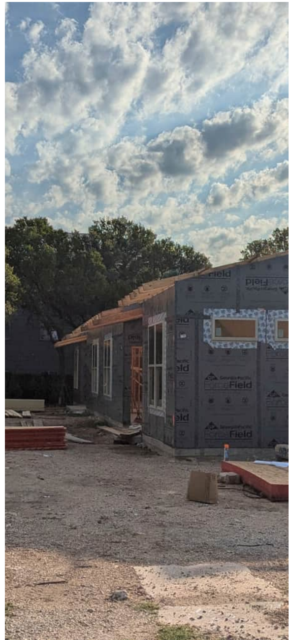
Duplex construction at 1106 Chestnut Street.
