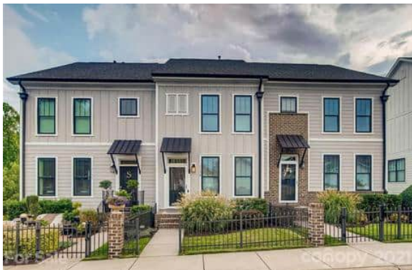
Traditional architectural style with moderate setbacks and front yard spaces.
