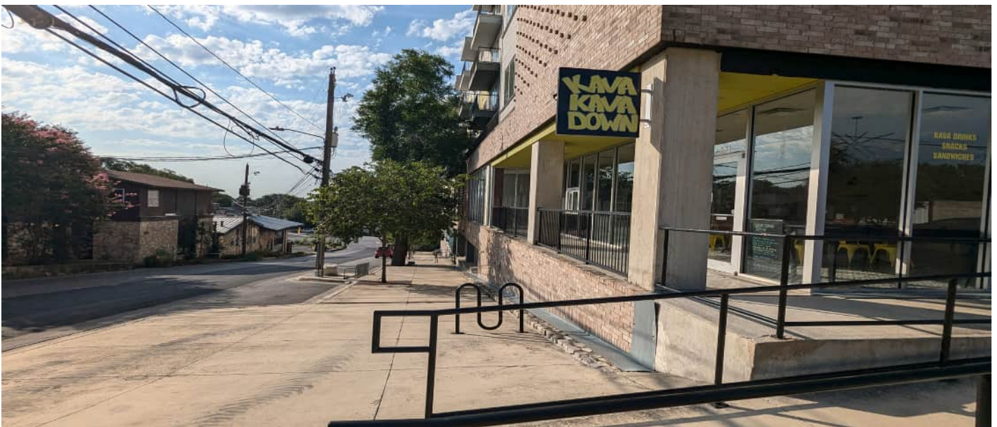
Vie Lofts' Commercial Space, 817 Chestnut Street.
