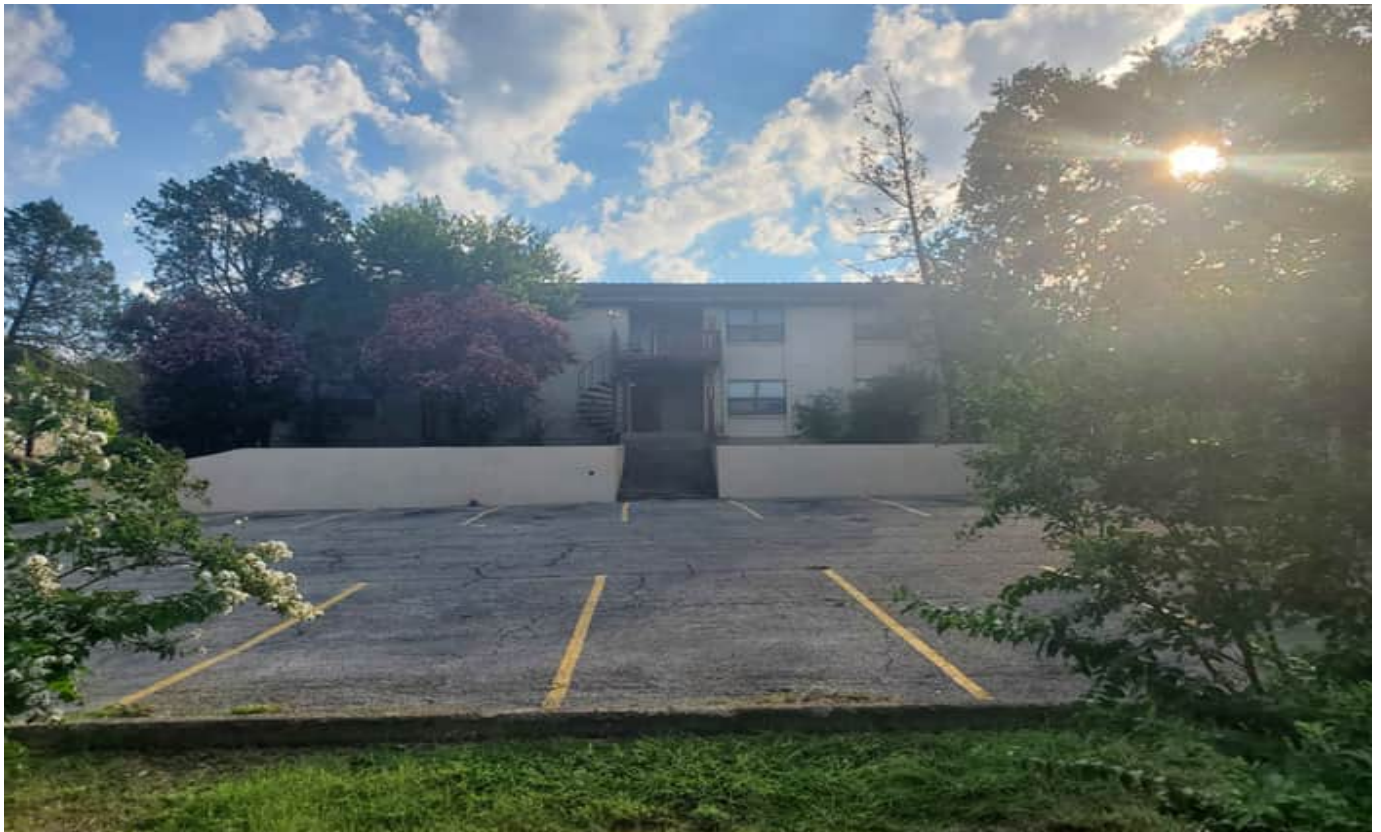
906 N LBJ Apartments with large street loaded parking lot and steep topography
