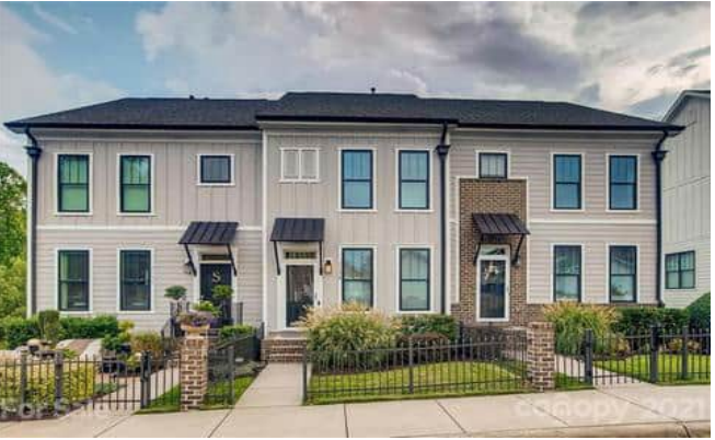
Traditional architectural style with moderate setbacks and front yard spaces.
