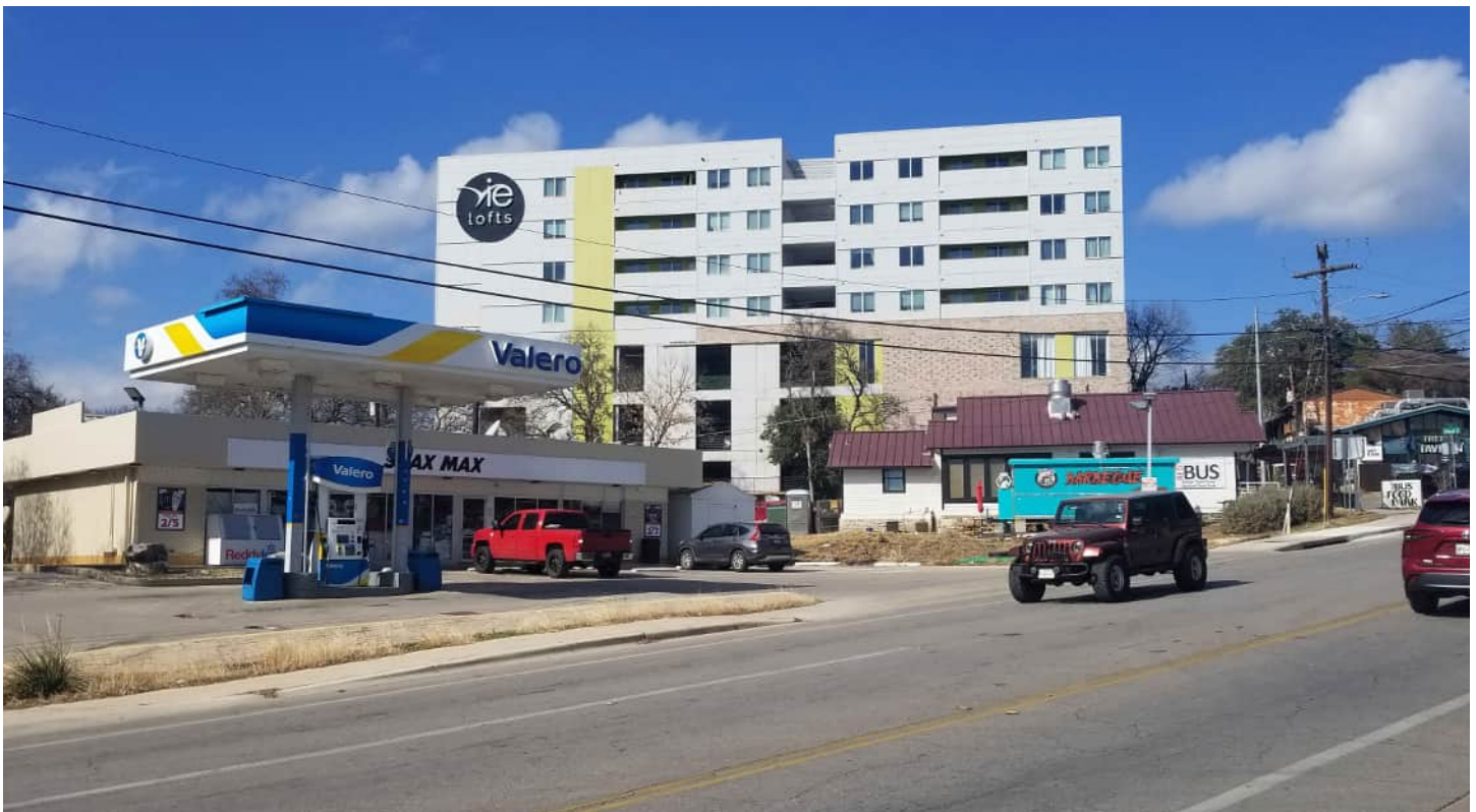
View the N. LBJ Drive Streetscape from the intersection of North LBJ Drive and Sessom Drive.
