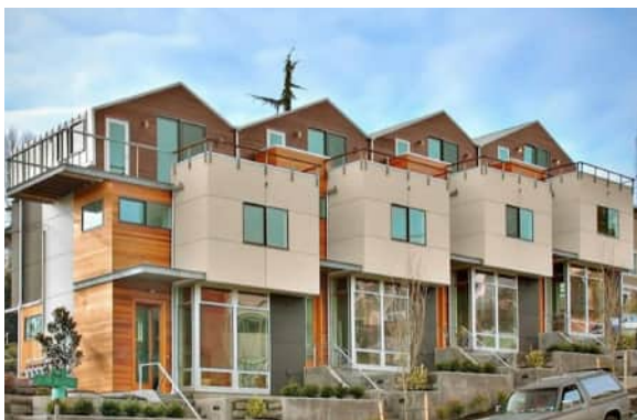
High transparency on ground floor, but offset in height from pedestrians on the sidewalk.
