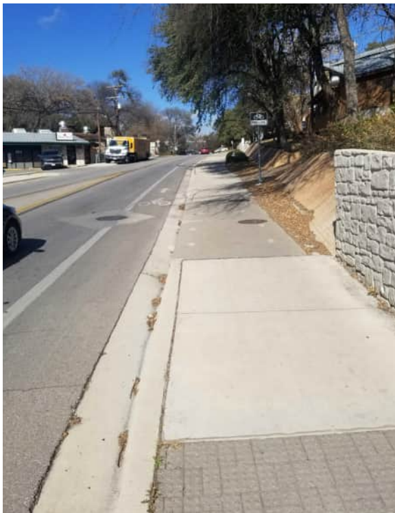
Newly improved sidewalk network along N LBJ Drive.
