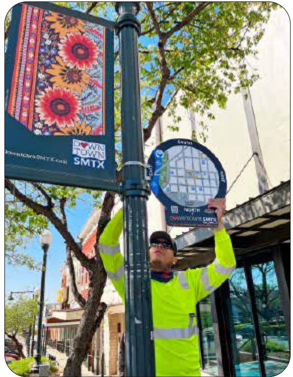
Wayfinding signs being installed Downtown (COSM)
