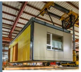
One "block" of a MiCASiTA modular home under construction. This component can become a 576-square foot standalone home, or multiple blocks can be combined to form a larger structure.
