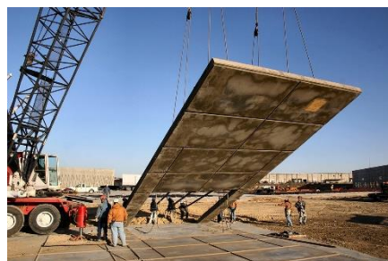
Concrete Tiltwall – may be precast or cast on site
