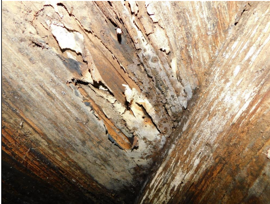
Girder separation, exterior load bearing concrete wall damage and black mold in crawl space
