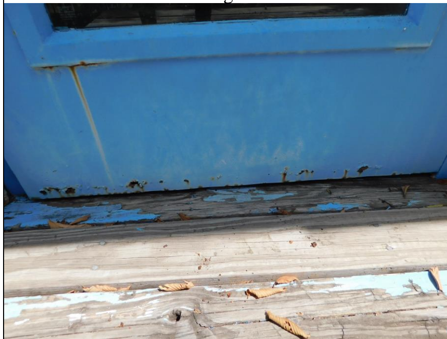
exterior door rust damage
