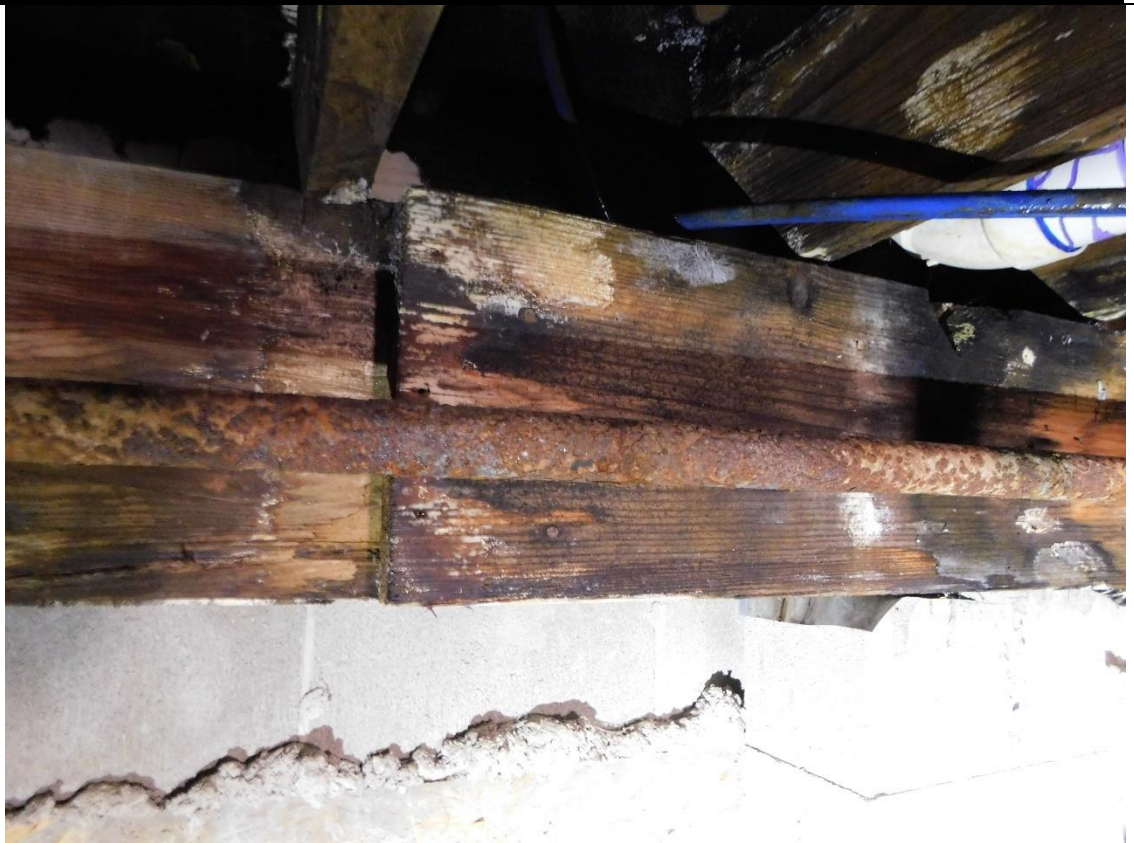
Girder separation, exterior load bearing concrete wall damage and black mold in crawl space
