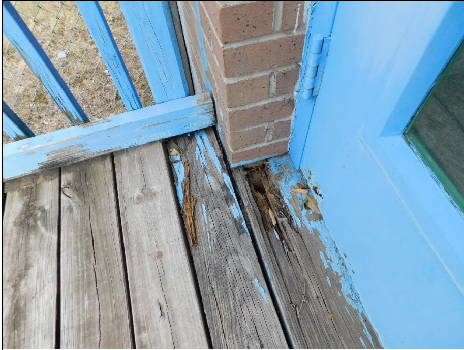
decking damage
