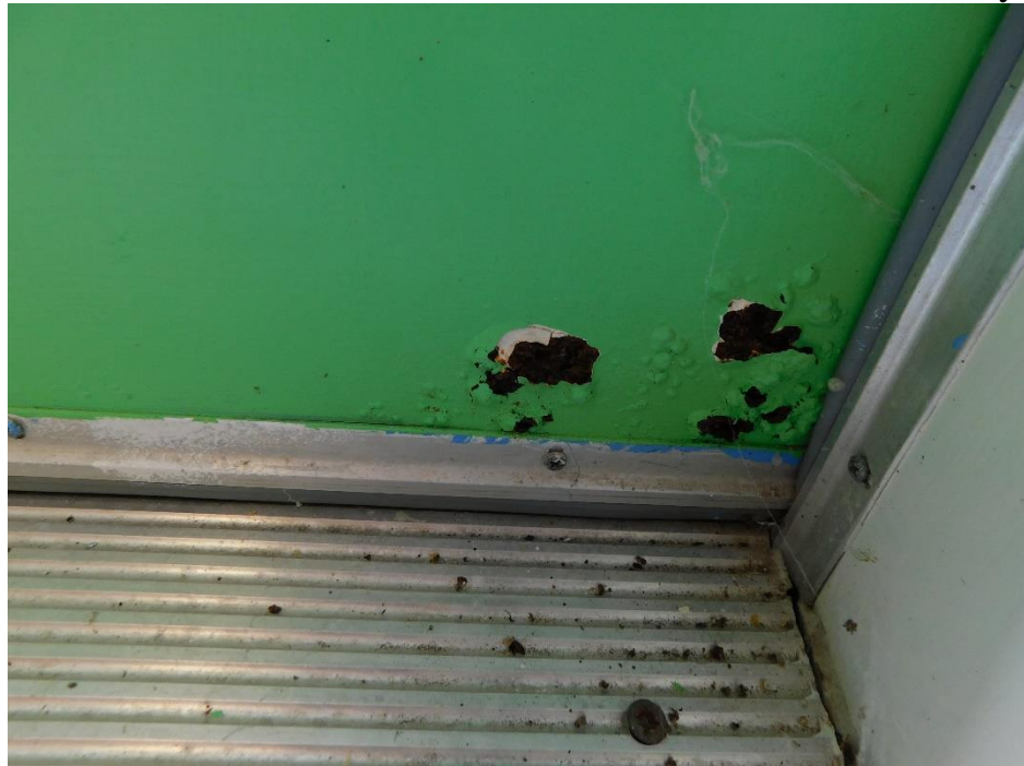
exterior door rust damage
