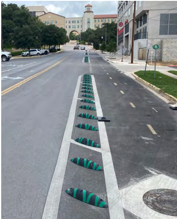
Cycle Track along Guadalupe Street
