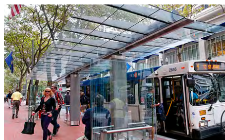
Prominent transit access and comfortable facilities
