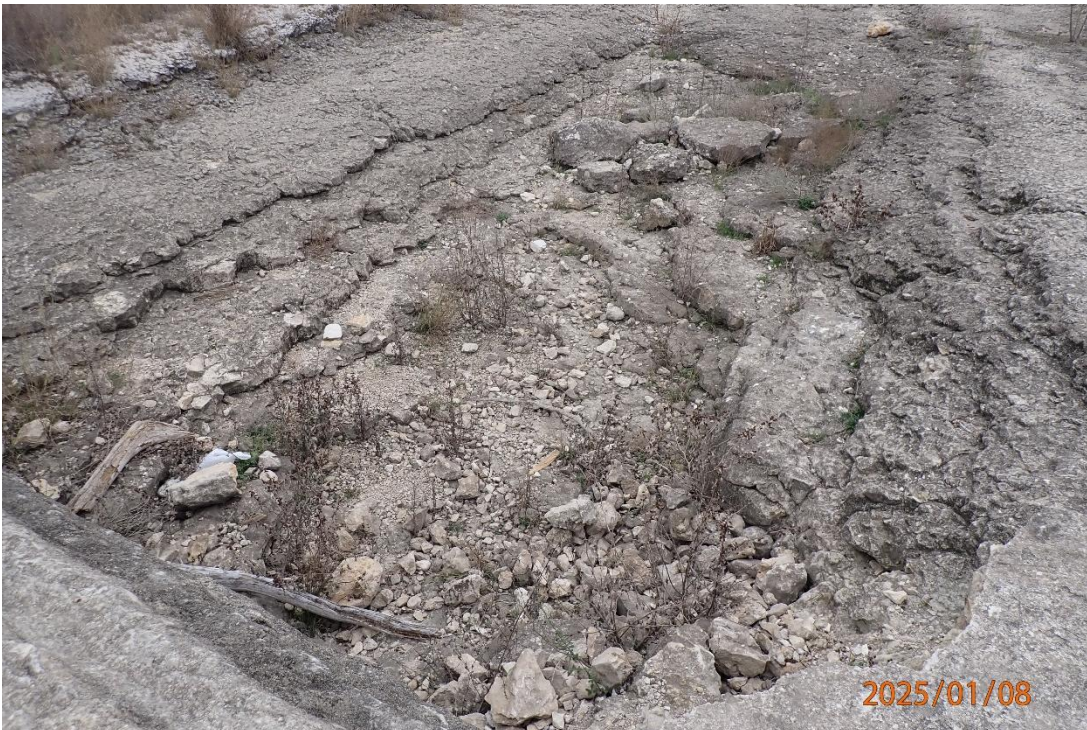
Photo No. 20: Looking downstream at scour hole
