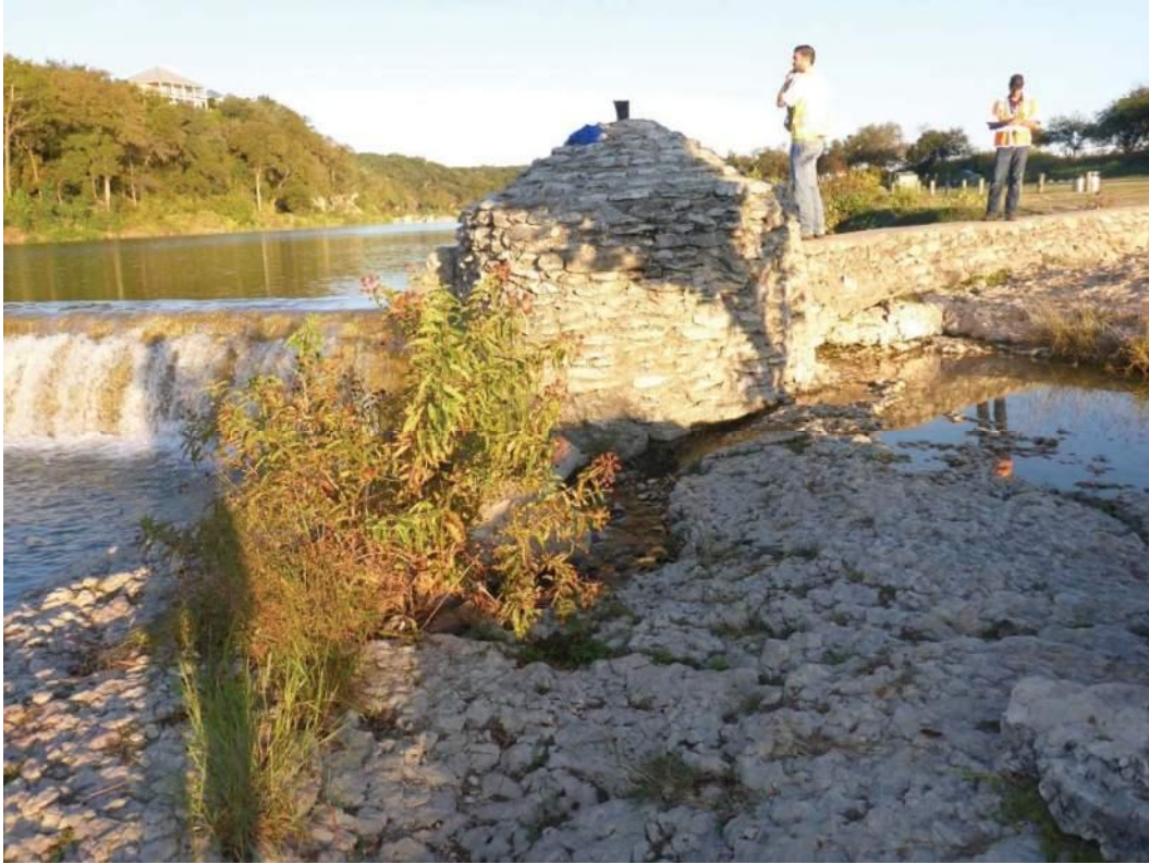
Photo 5 – Seep at Left Abutment
