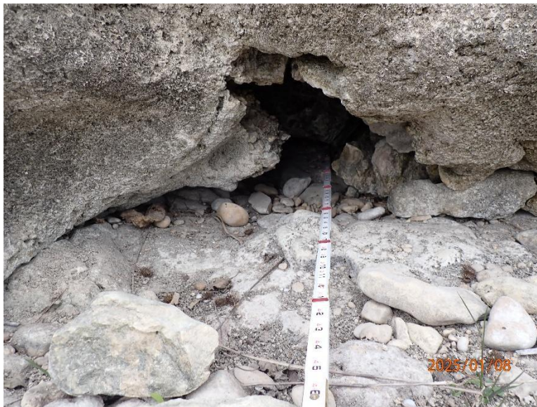
Photo No. 8: 2' to 3' deep voids on downstream toe
