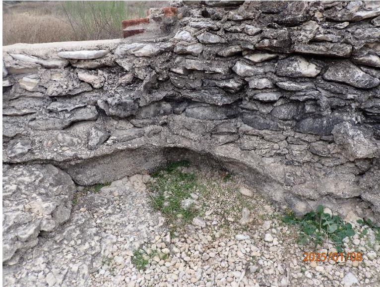
Photo No. 2: Scour erosion on upstream side of left abutment
