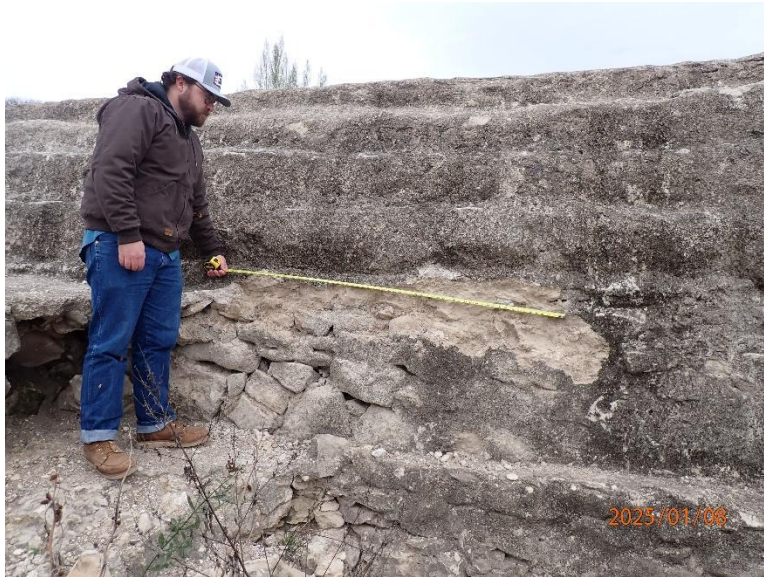
Photo No. 7: 5-foot-wide broken off section on downstream face
