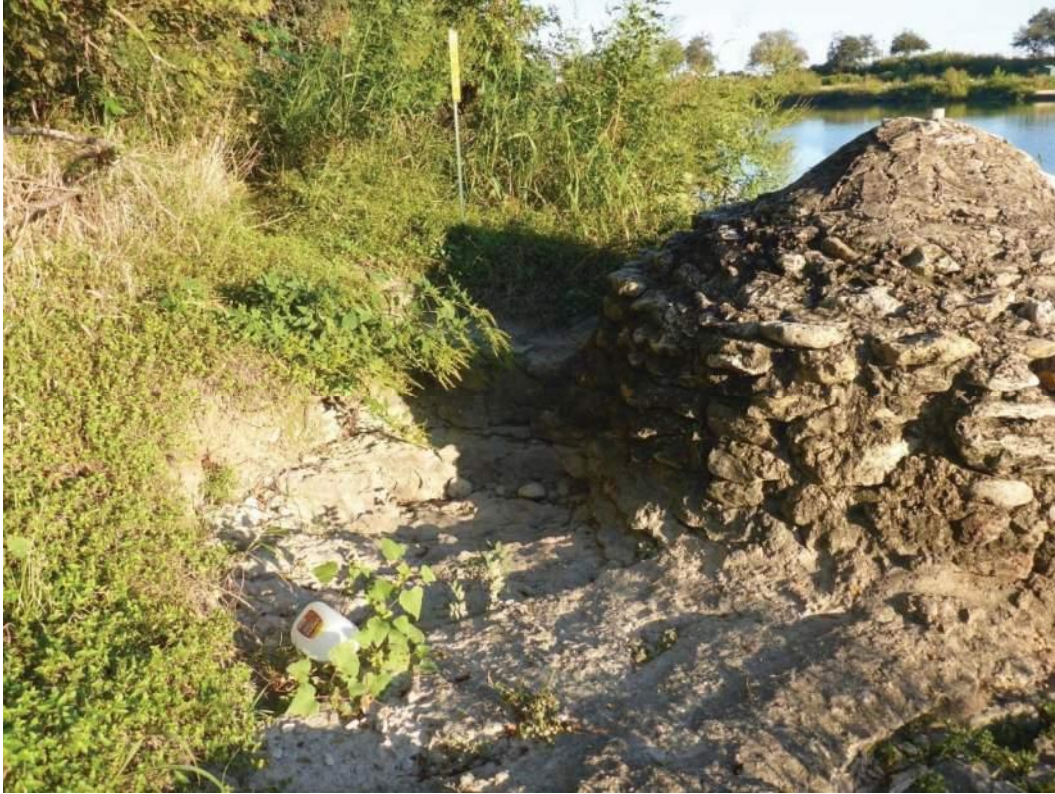
Photo 9 – Pocket of Erosion at Groin Downstream of the Right Abutment
