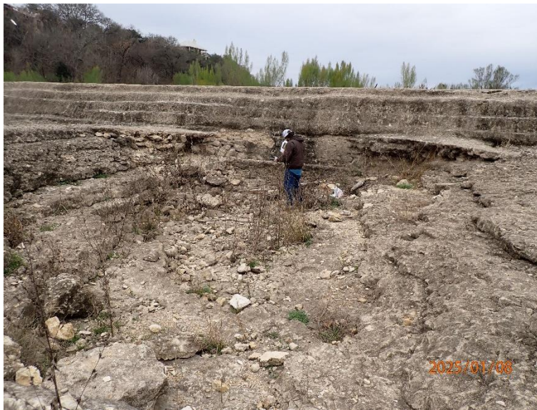
Photo No. 6: 22-foot-wide scour on the downstream face
