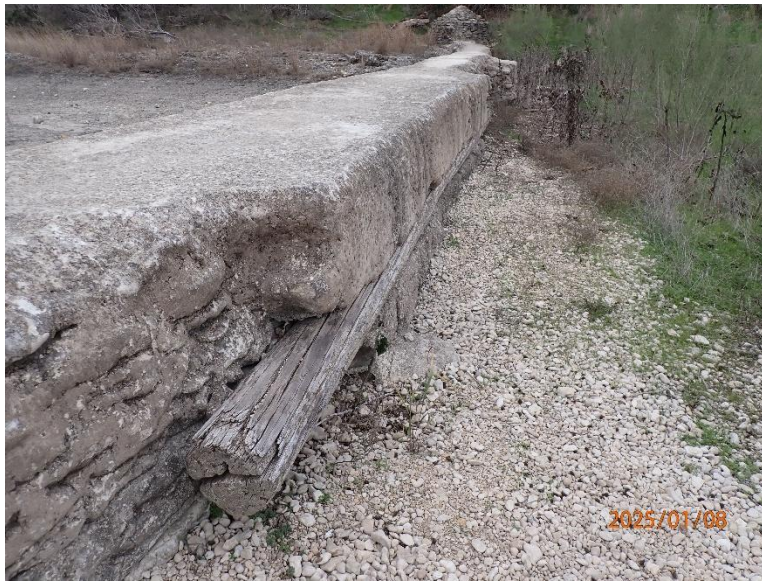
Photo No. 4: Log embedded on the upstream face
