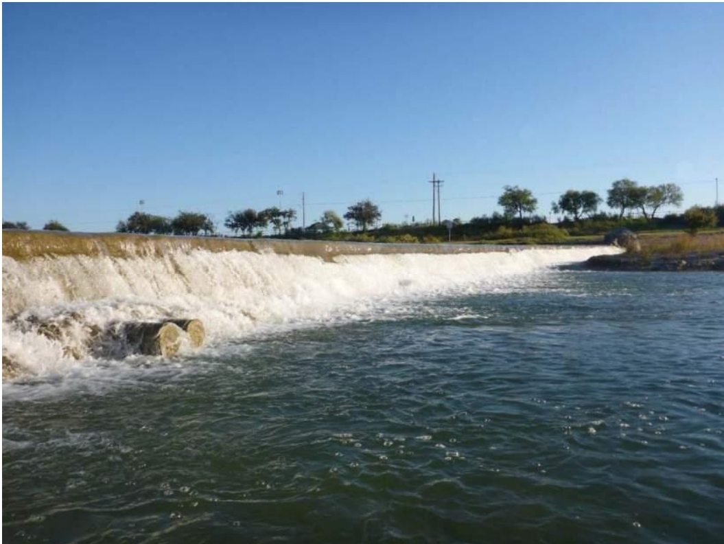
Photo 10 – Low-Flow Outlet Pipes with Infill Concrete
