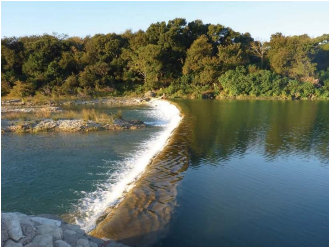
Photo 2 – Crest of the Dam (Primary Overflow Section)
