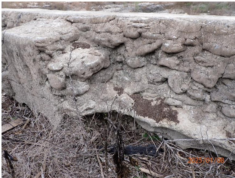
Photo No. 5: Minor scour on upstream toe
