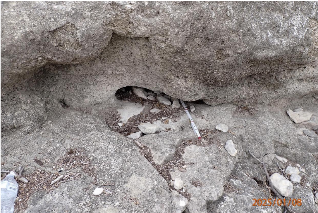
Photo No. 18: Void on downstream toe
