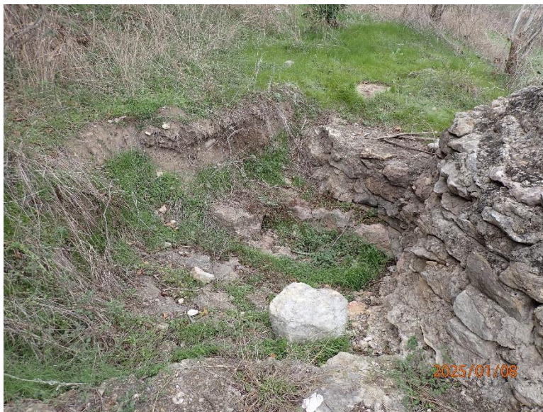
Photo No. 3: Eroded section at the right abutment
