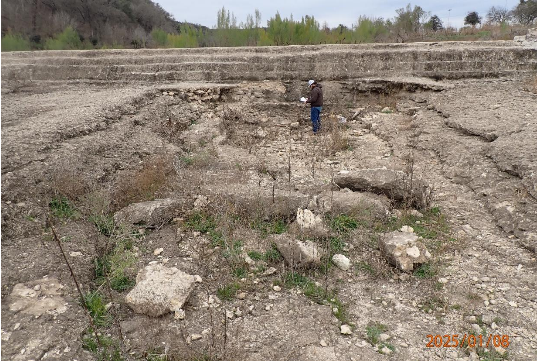
Photo No. 19: Scour on downstream toe
